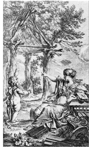
Figure 2.6: Frontispiece of Marc-Antoine Laugier: Essai sur l’architecture 2nd ed. 1755 by Charles Eisen (1720–1778). Allegorical engraving of the Vitruvian primitive hut.
