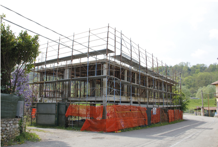
FIGURE 2.3.6 - GURONE MILLS. BUILDING UNDER CONSTRUCTION
