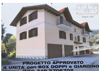
FIGURE 2.3.19 - PHOTO FROM THE SITE
