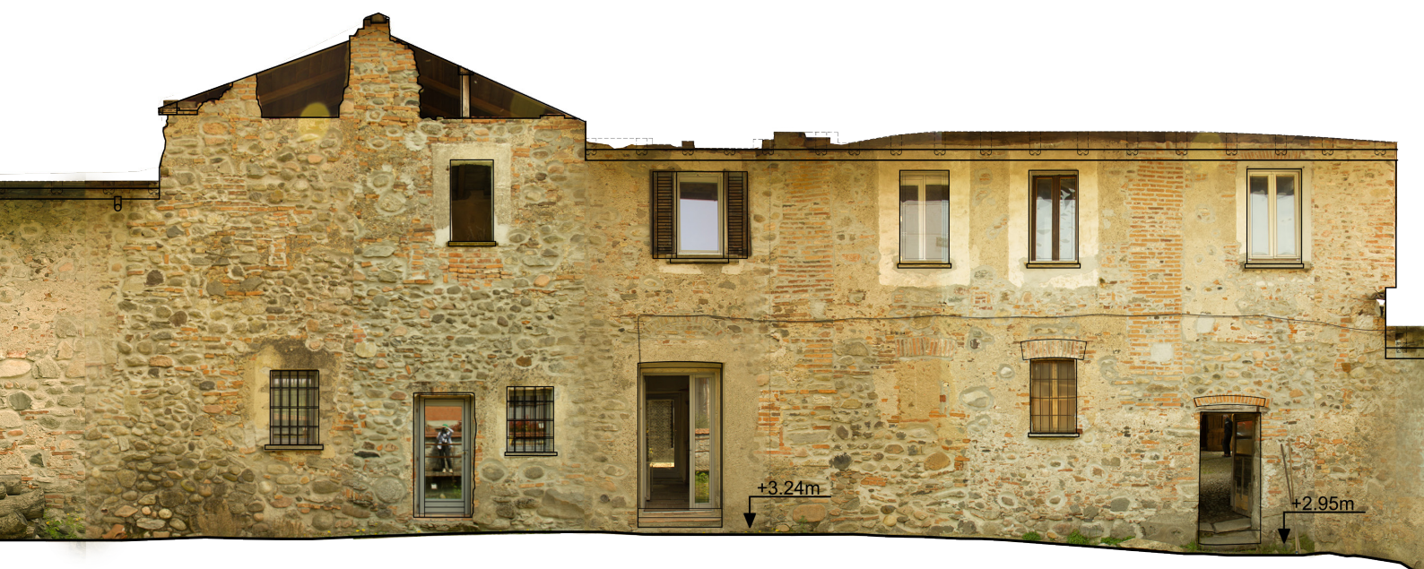
Figure 4.4.5 - Canal. Longitudinal elevation rectified imagery in scale 1:100
