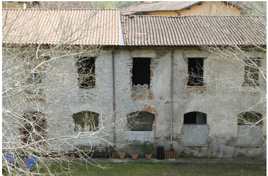
FIGURE 2.3.7 - GURONE MILLS. BUILDINGS UNDER RENOVATION
