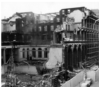
FIGURE 2.3.16 - DEMOLITION OF THE GENERAL POST OFFICE BUILDING IN MANCHESTER, APRIL 1967. SOURCE: NP ESTATES, LOST BUILDINGS OF MANCHESTER
