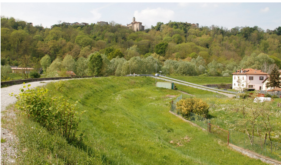
Figure 4.4.8 - Site visit photos of the area that presents inconsistency in DTM
