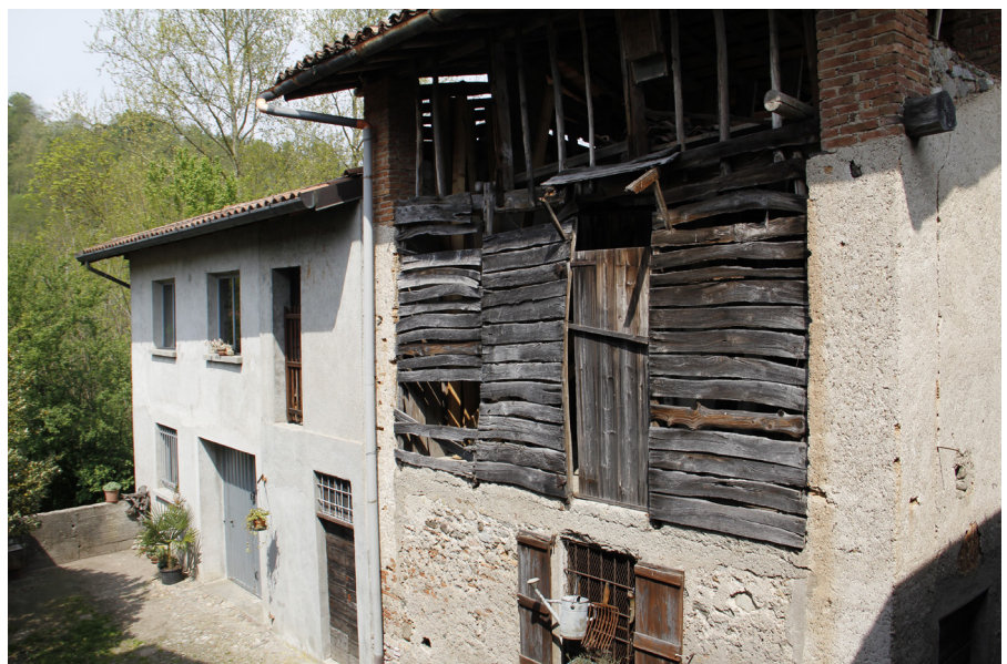
FIGURE 2.3.7 - GURONE MILLS. ABANDONED BUILDING
