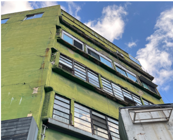
The original section built in 1937, the portion added during the 1962 extension, and the area appended as a result of the 1978 road expansion project can all be seen simultaneously.
