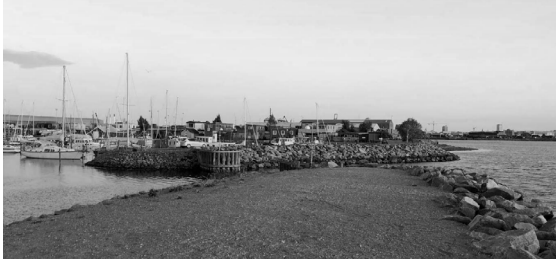
Figure 5.14 Current condition of Skudehaven Lake. Source: Author's photograph.
