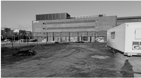
Figure 5.15 Current condition of Nordhavn Metro Station. Source: Author's photograph.
