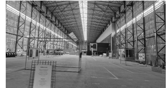
Figure 5.8: Current condition of Tunnelfabrikken Source: Google Maps.
