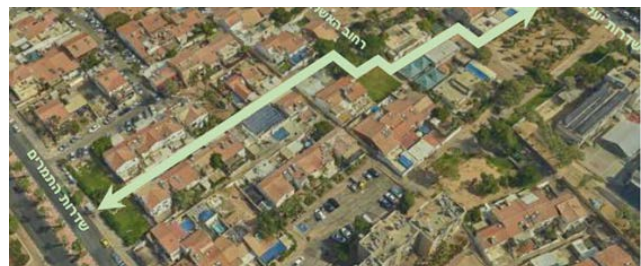
Figure 118. Independent Houses block. Source: Eilat's Municipality
