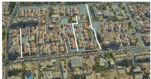
Figure 117. Independent Houses block. Source: Eilat's Municipality
