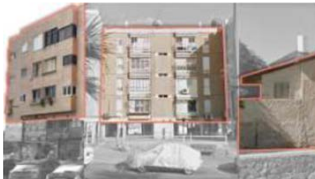
Figure 129. Typical facade with “Eilat Stone”, Source: Eilat’s Municipality
