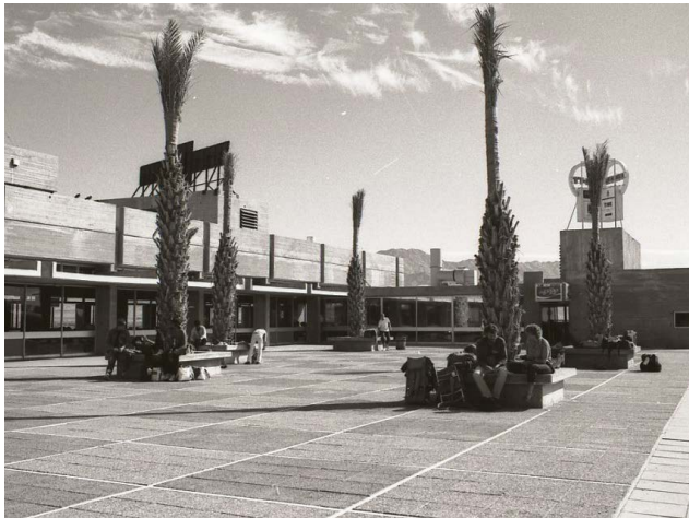
Figure 163. Central Bus station, 1981. (Source: National Library of Israel)
