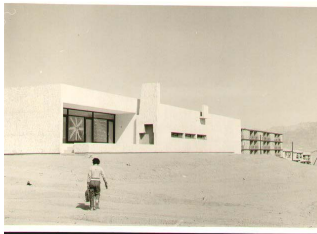
Figure 179. Community Centre, 1967 Source: Eilat Archive
