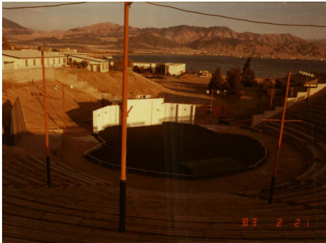
Amphitheatre Renovation, 1983. (Source: Eilat's archive)
