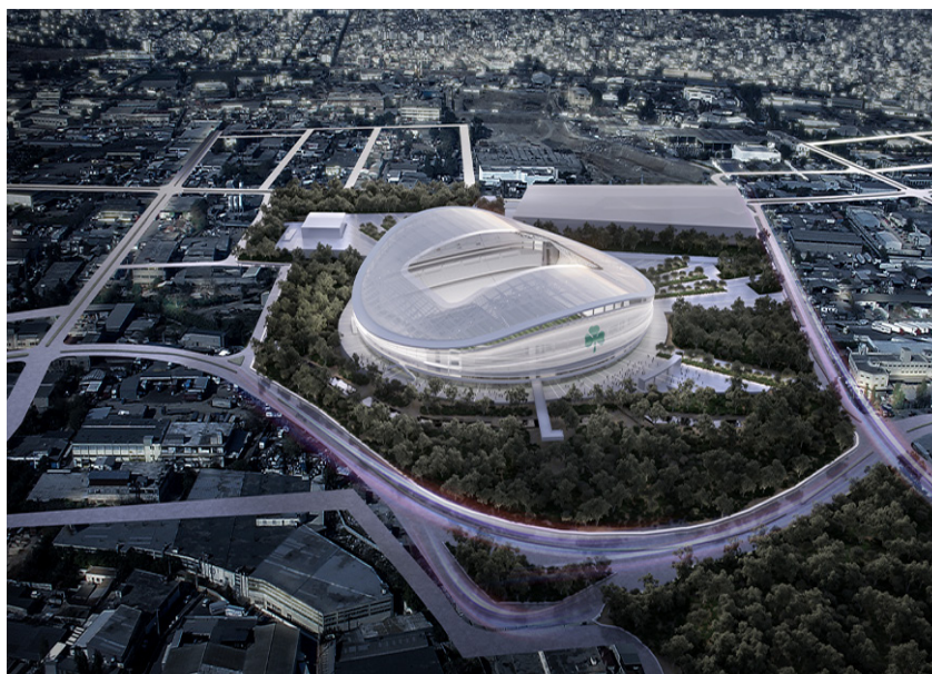
Figure.18 Title:PAO's Stadium, Double regeneration program Source: A&A ARCHITECTS' Archive
