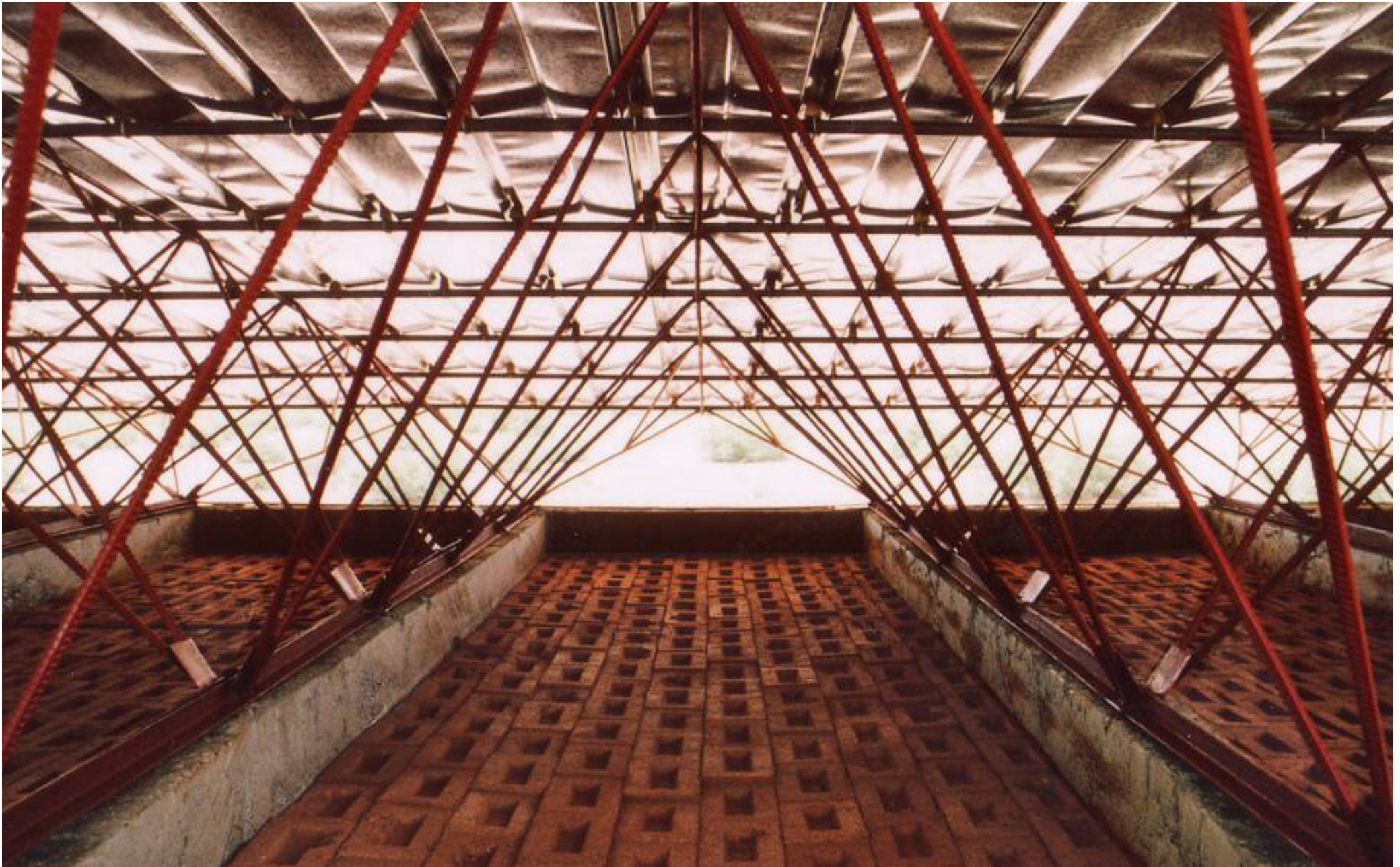
Figure 69: Roof of Gando primary school Diébédo Francis Kéré
