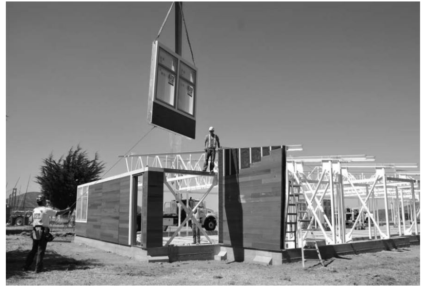
Figure 59: Panel lifting
