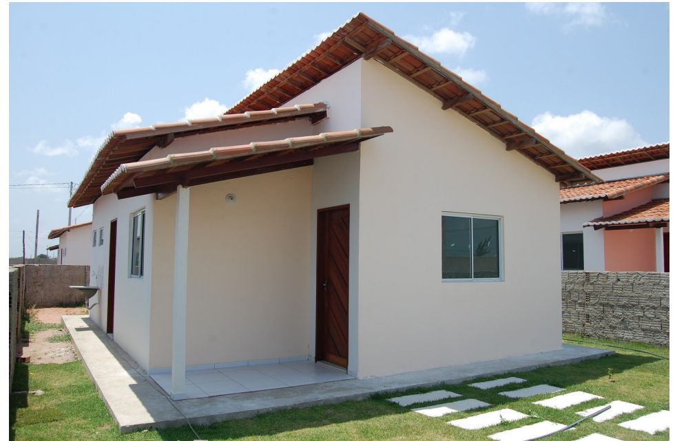
Figure 23: Typical brick and concrete house
