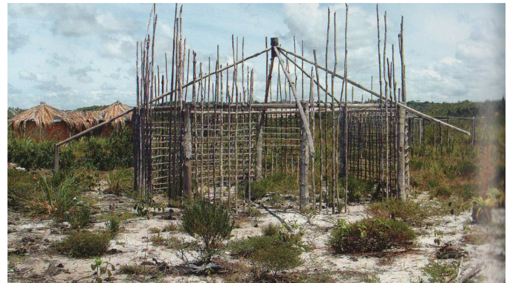
Figure 21: Timber structure to receive the compact mug
