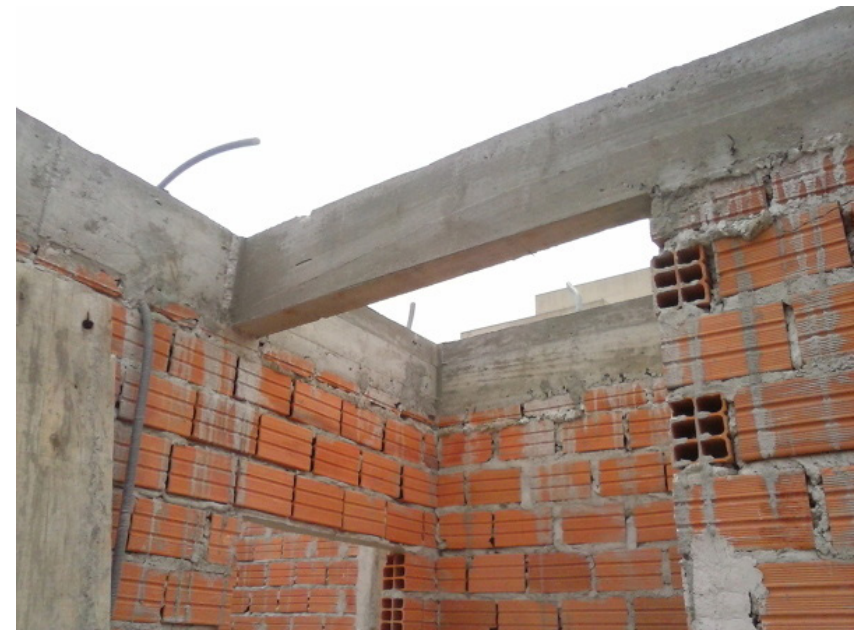
Figure 22: Concrete post and beam structure and brick wall
