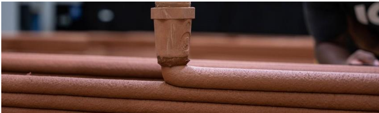
Figure 54. Additive construction of Mars Dune Alpha.
