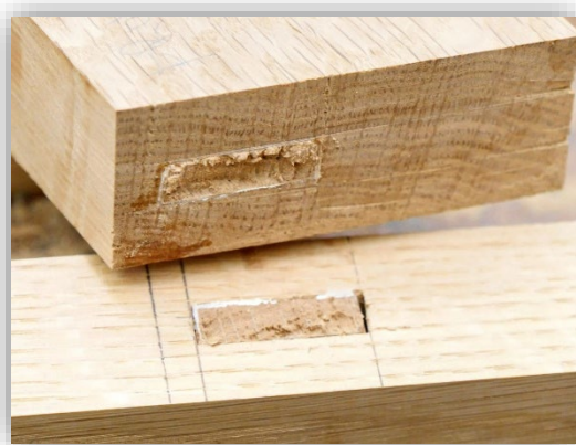
Figure 7. Failed mortise and tenon joint
