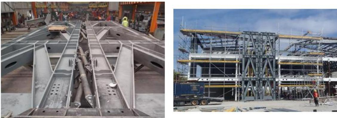
Figure 2-31: Left: pair of steel braced frames assembled in the workshop with dampers; right: pair of steel braced frames erected on-site [93]
