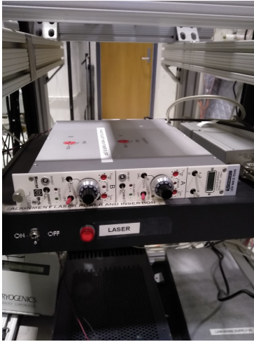
Figure 4.10: dual high voltage supply unit
