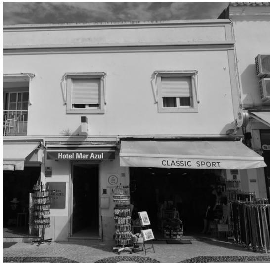
fig. 24 Rua 25 de April shops_2 Site survey
