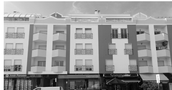
fig. 20 Residential building Avenida dos Descobrimentos Site survey
