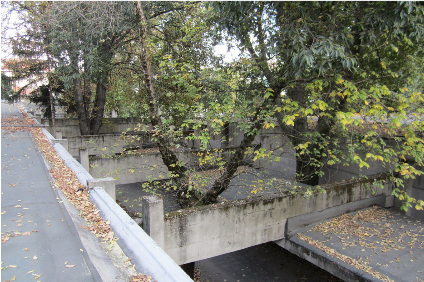
Main pathway View of roof from top
