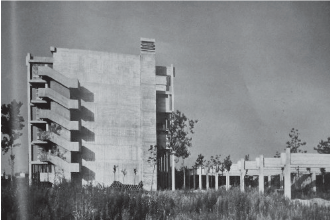
Reformatory dwellings Side facade with exterior staircase
