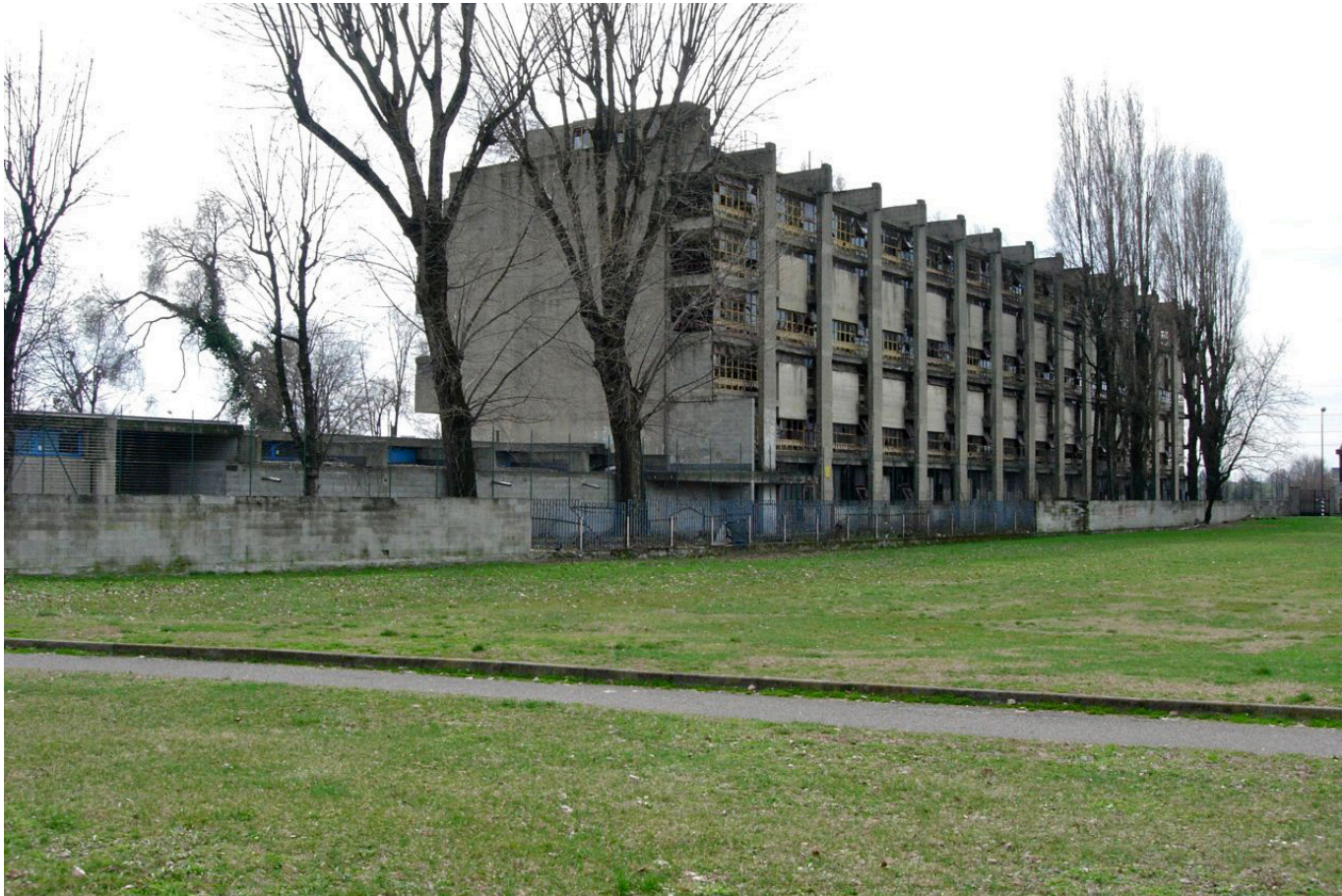
Reformatory dwellings Back facade
