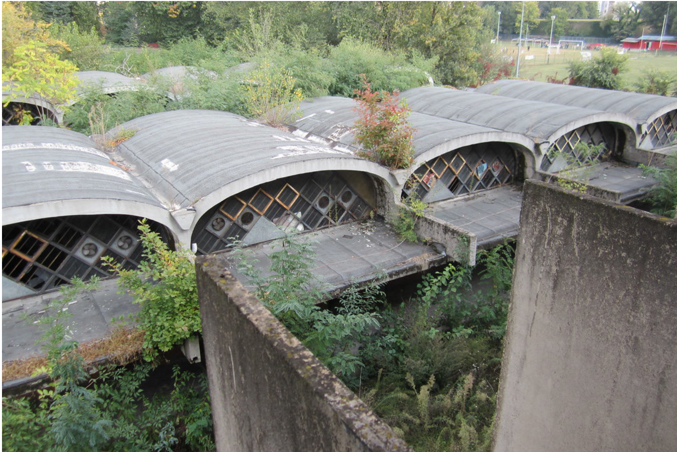
Elementary school Back facades
