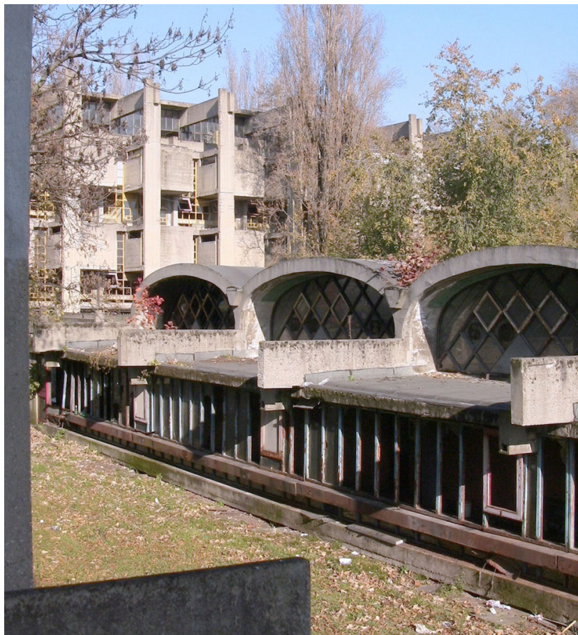
Elementary school Back facade, with reformatory dwellings (center back)
