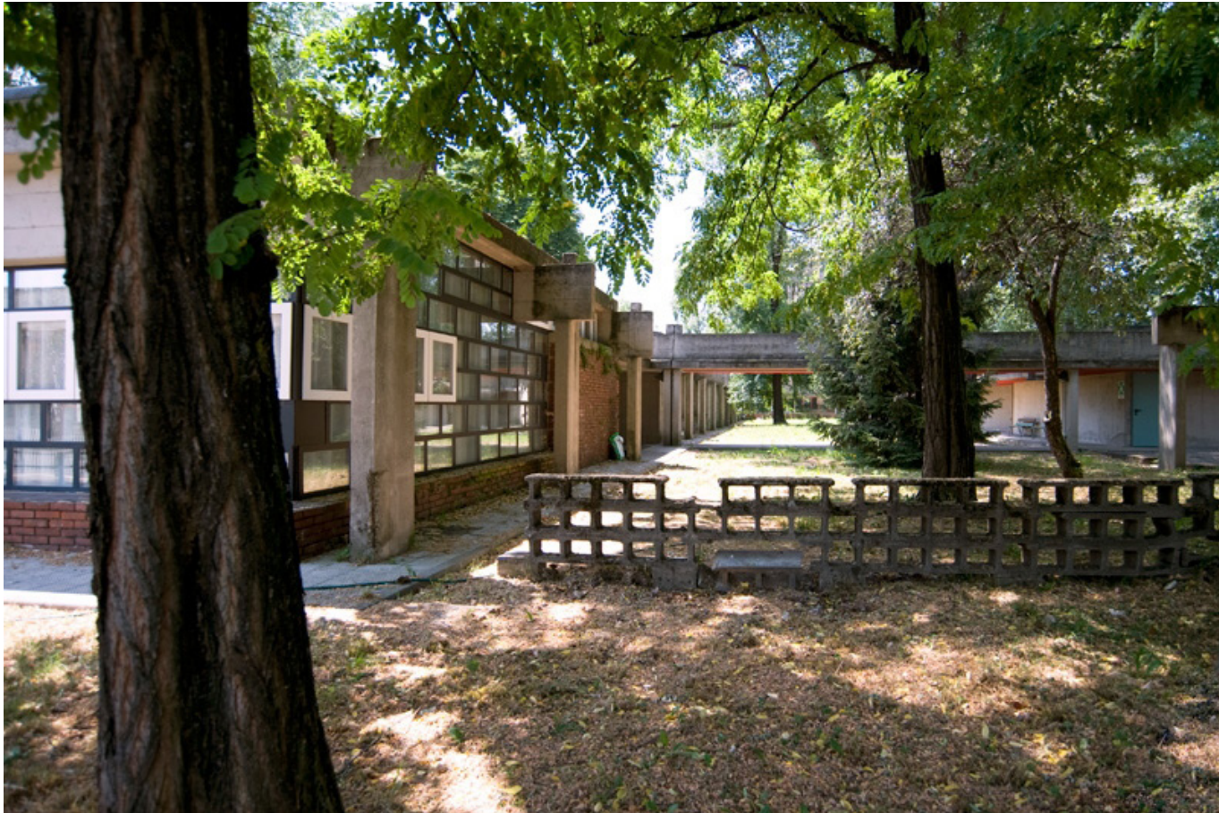
View of the guesthouse and courtyard.
