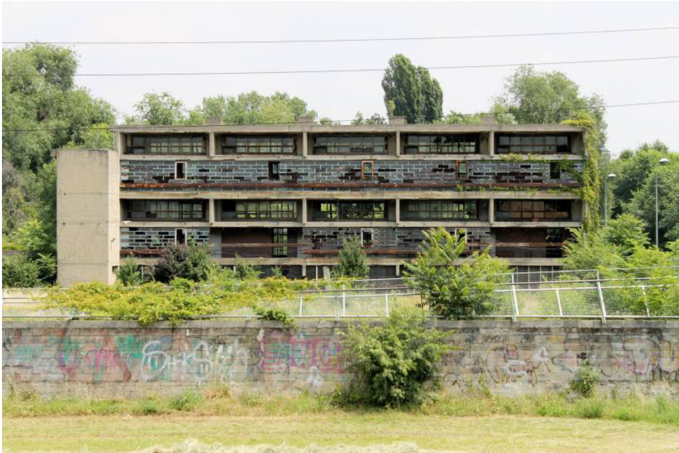
Middle school Back facade
