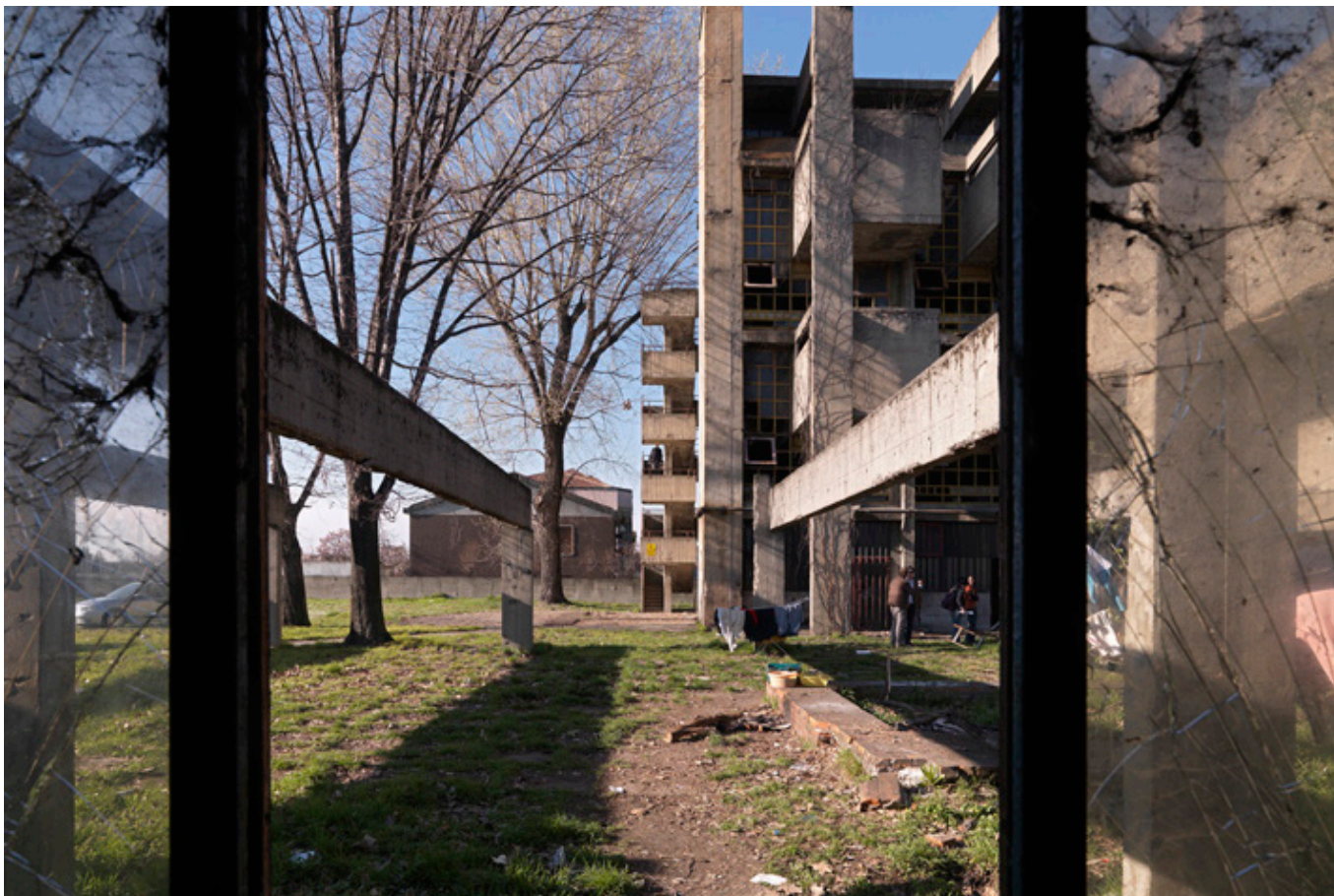
Reformatory dwellings Front facade and external staircase
