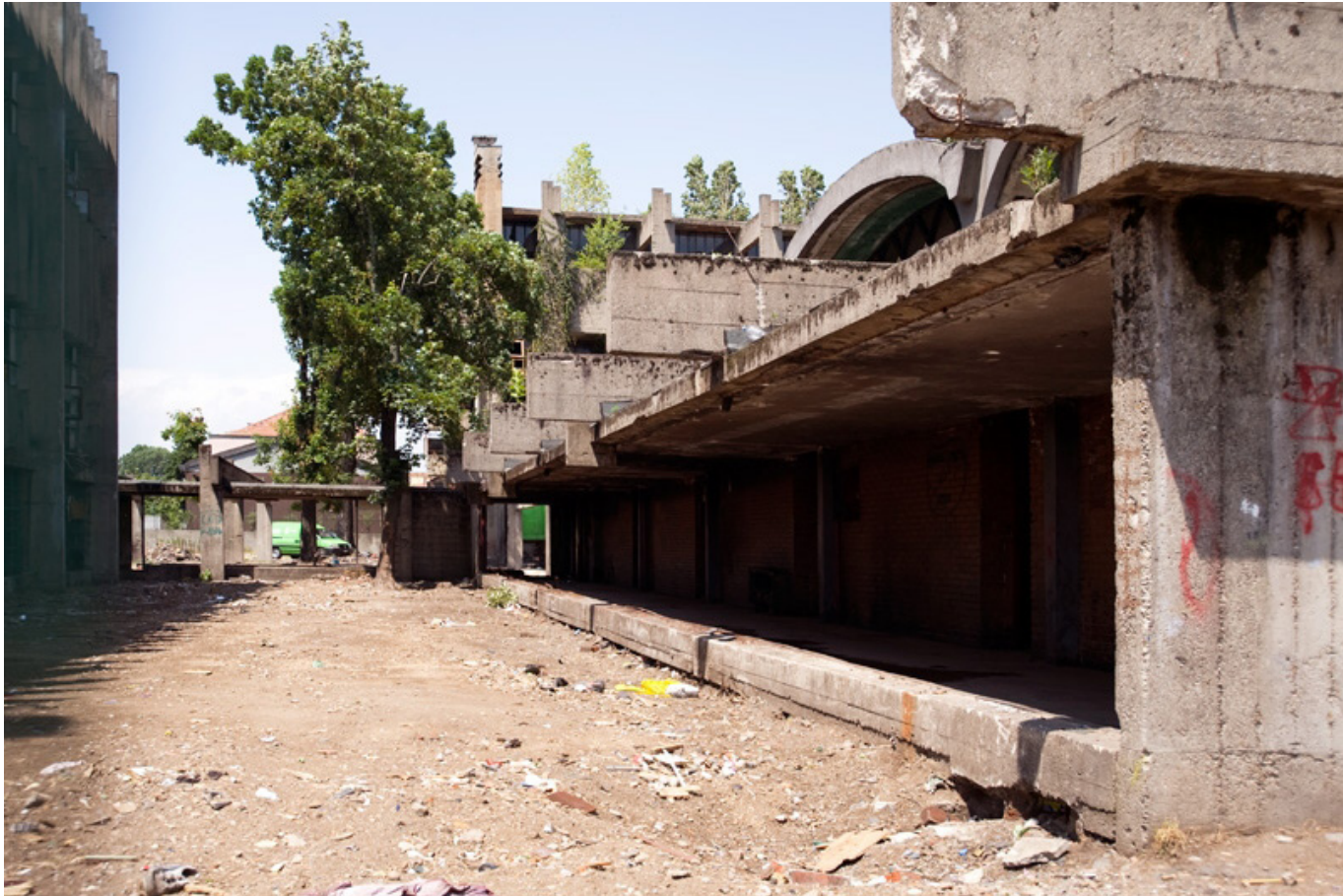
Elementary school Back facade
