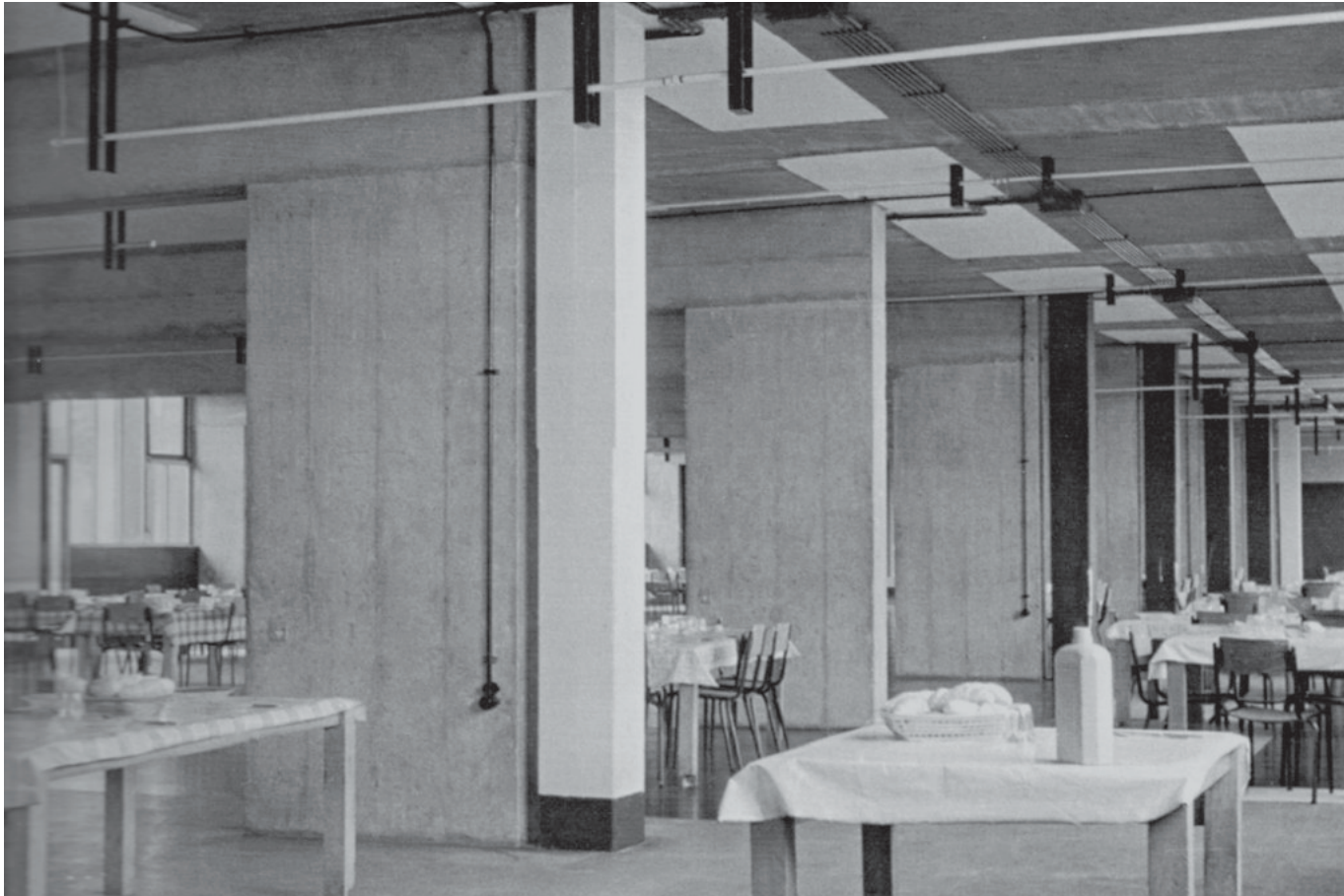
Reformatory Dwellings Main cafeteria at ground floor
