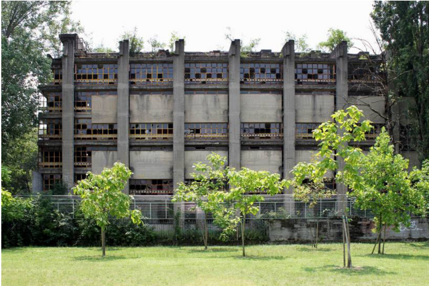
Reformatory dwellings Back facade
