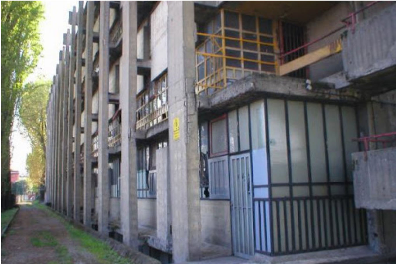
Reformatory dwellings Back facade
