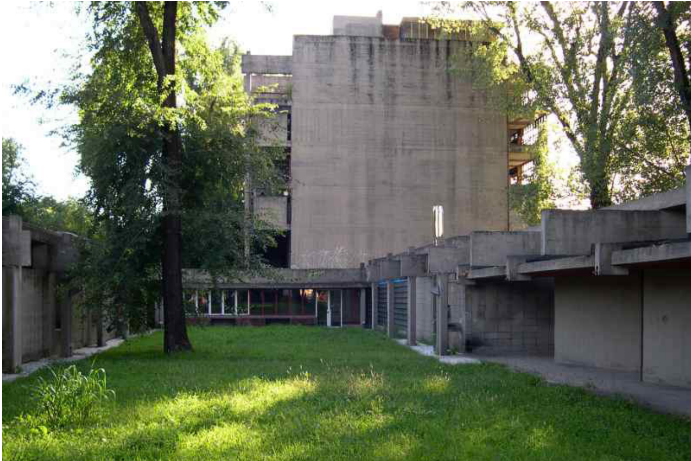
Reformatory dwellings Side facade and services buildings
