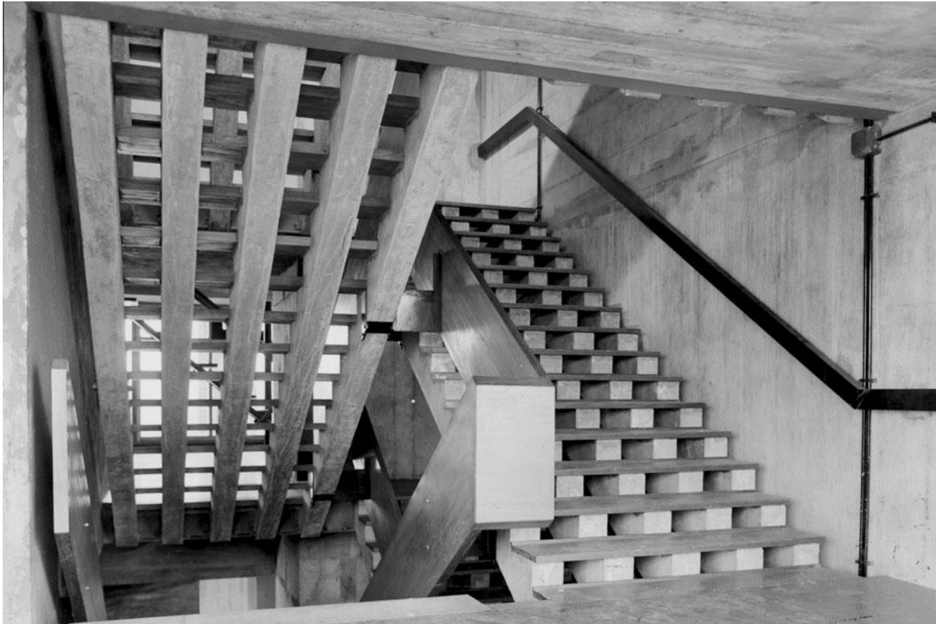
Reformatory dwellings Main staircase, intermediate floor
