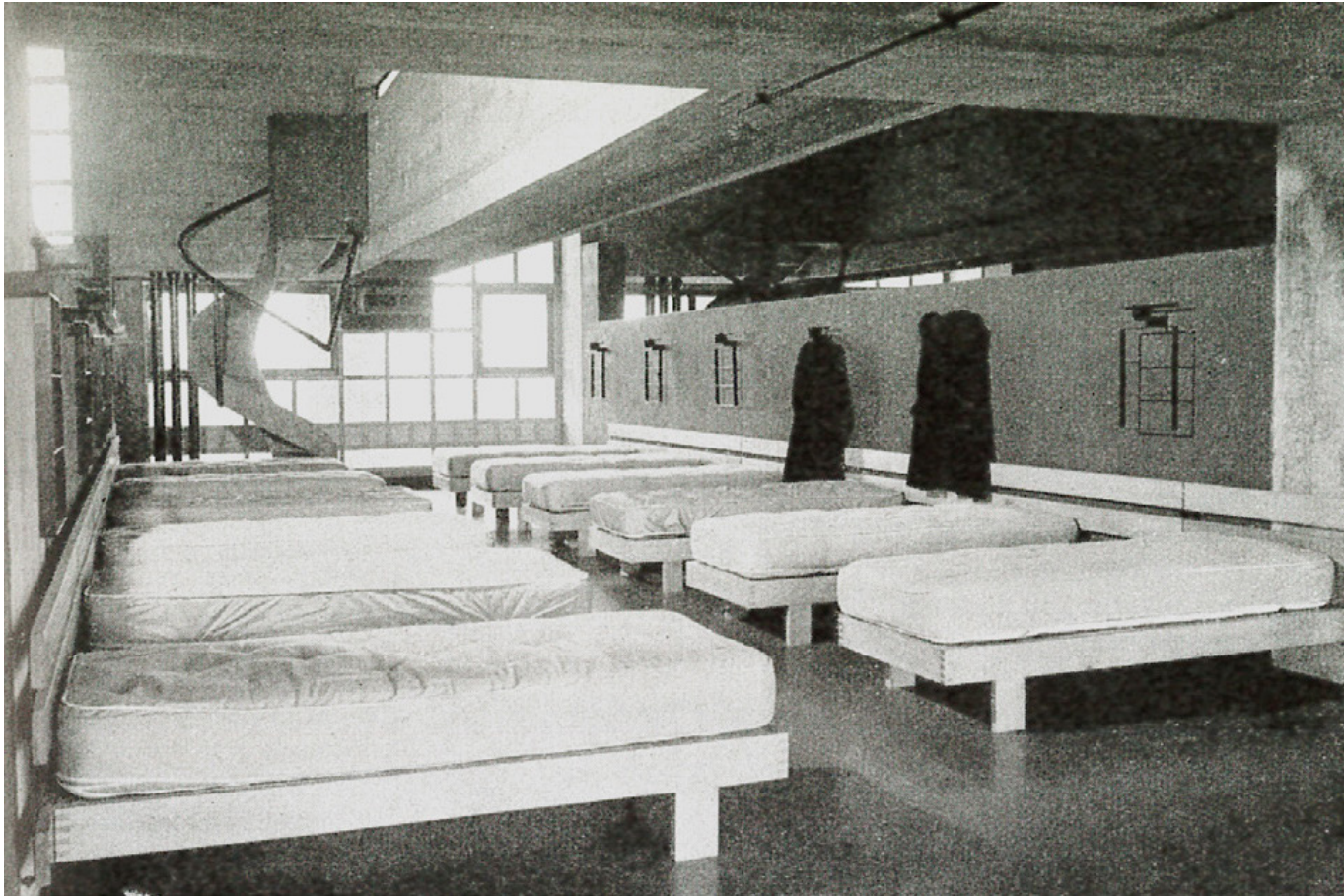
Reformatory dwellings Interior photograph of the dwelling units
