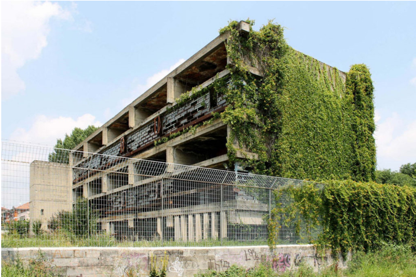
Middle school Back facade
