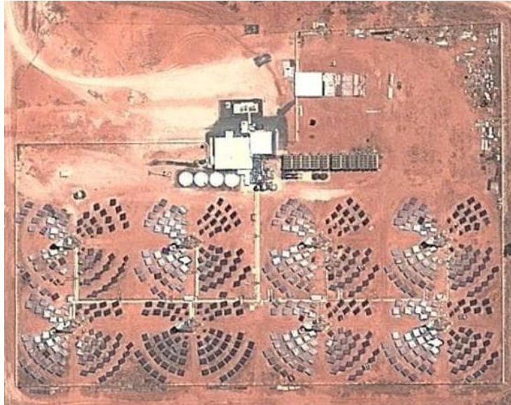
Figure 21 Lake Cargelligo power plant
