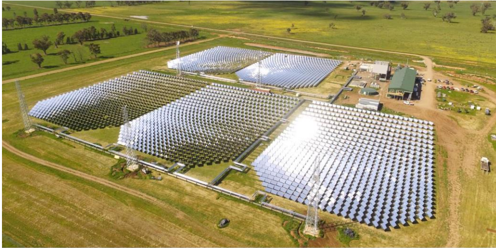
Figure 45 Aerial picture of Jemalong power plant
