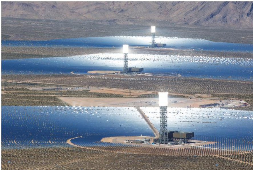
Figure 11 The Ivanpah Solar Electric Generating System
