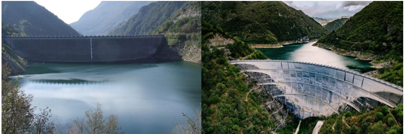
Figure 21: Ponte Cola, watershed and dam body detail (ProgettoDighe, 2021; GDB, 2020).
