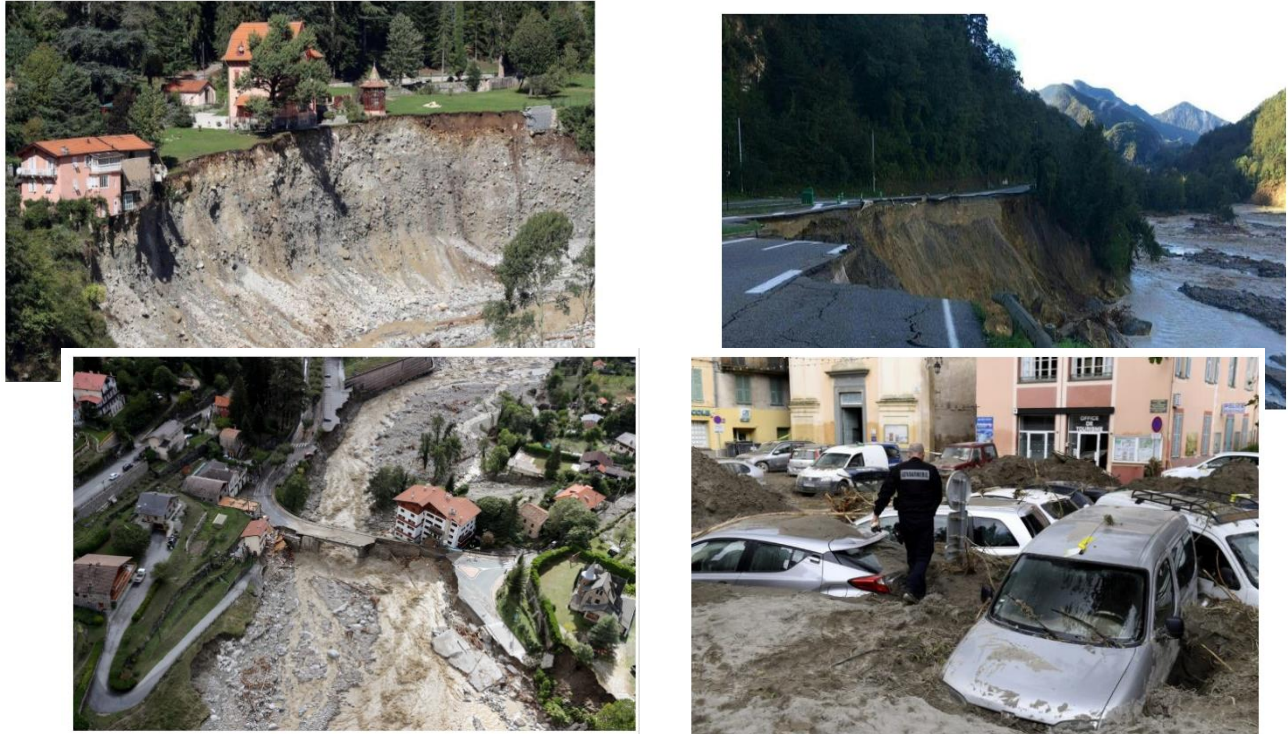
Figure 20: Landslide and Flooding due to Alex Storm (BBC)
