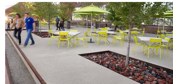
The steel on the edge of the coffee terrace and the tree pond comes from recycled old railroad tracks, and the tree pond is planted with maple trees and covered with recycled red brick rubble.
