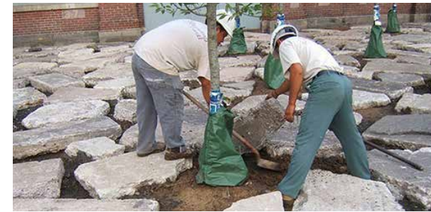
The previous material is used for the new pavement
