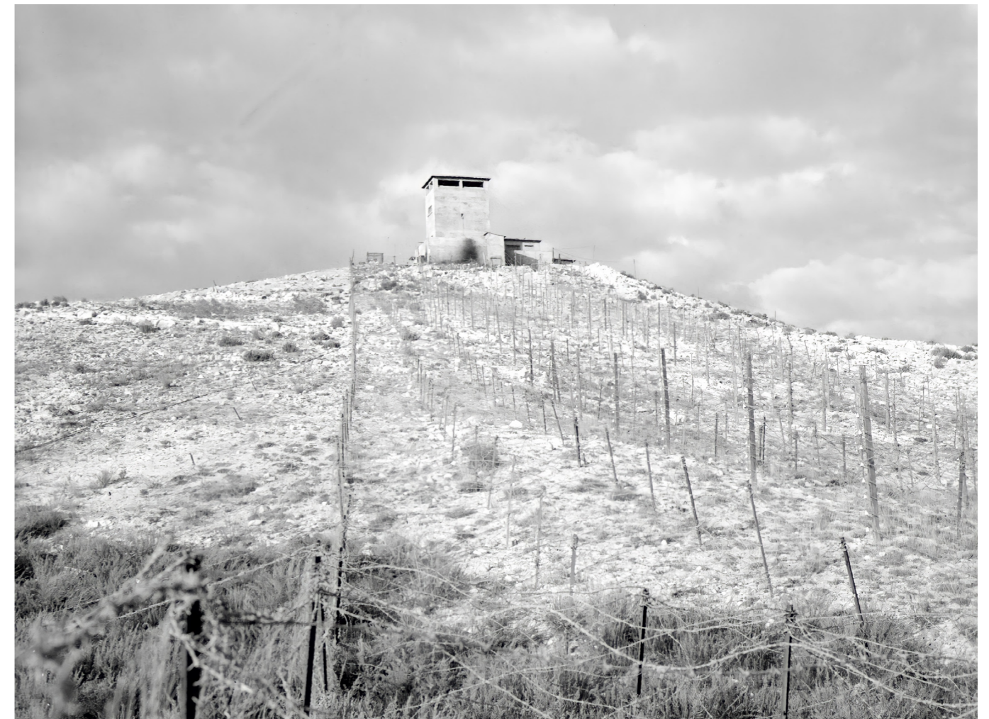
Fig. 7 The construction of the forbidden zones and the defensive line called Ligne Morice along the Algerian border with Tunisia, October 1959.
