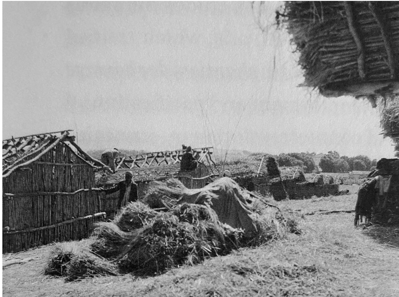
Fig. 8 Forcibly displaced people building shelters in the camp de regroupement of Taher El Achouet in Constantine, 1957.
