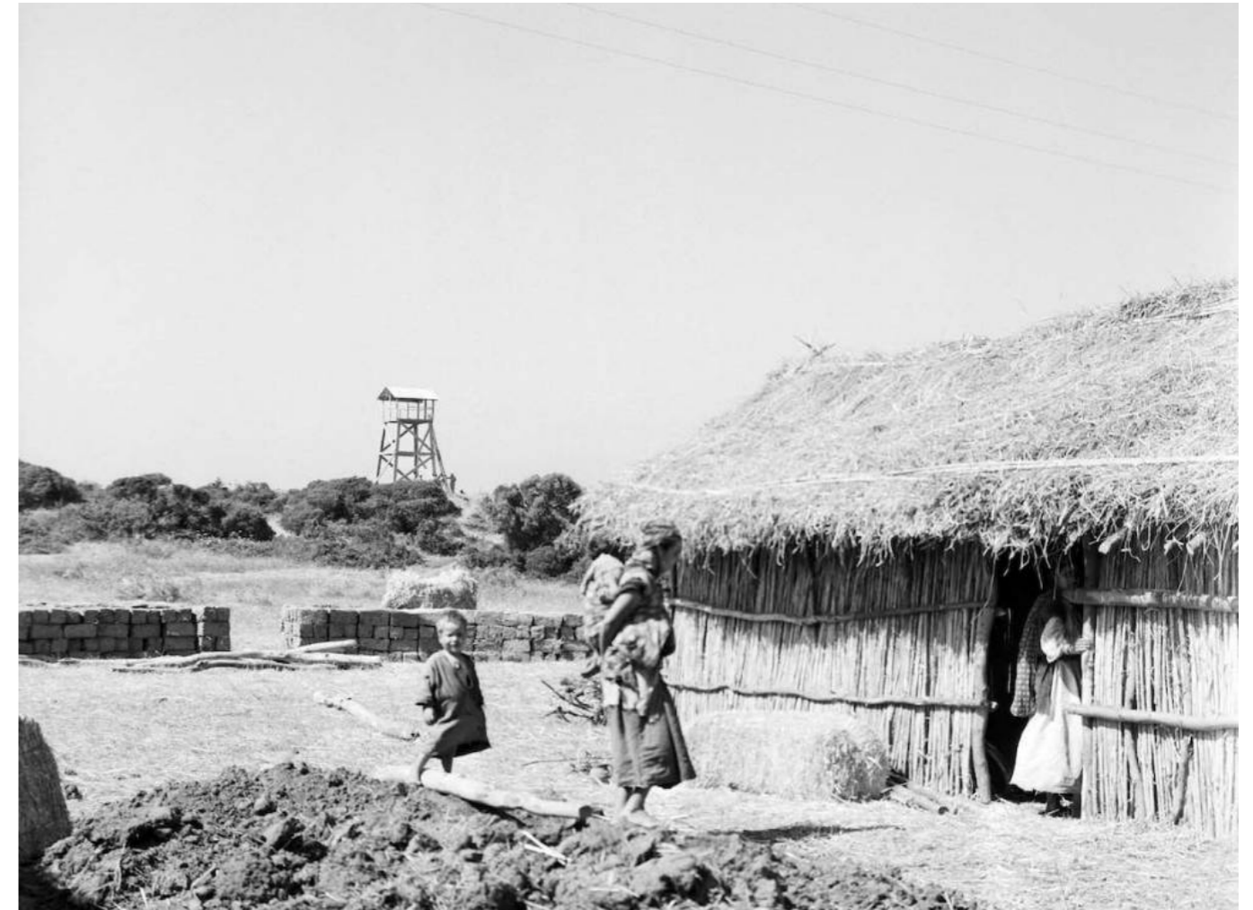
Fig. 9 Forcibly displaced people building shelters in the camp de regroupement of Taher El Achouet in Constantine, 1957.
