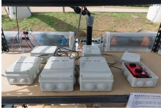
Figure 8-19: Data collectors of the IoT system with connection to sensors of Temperature and Humidity.
