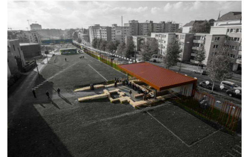
Construction of the Wall
