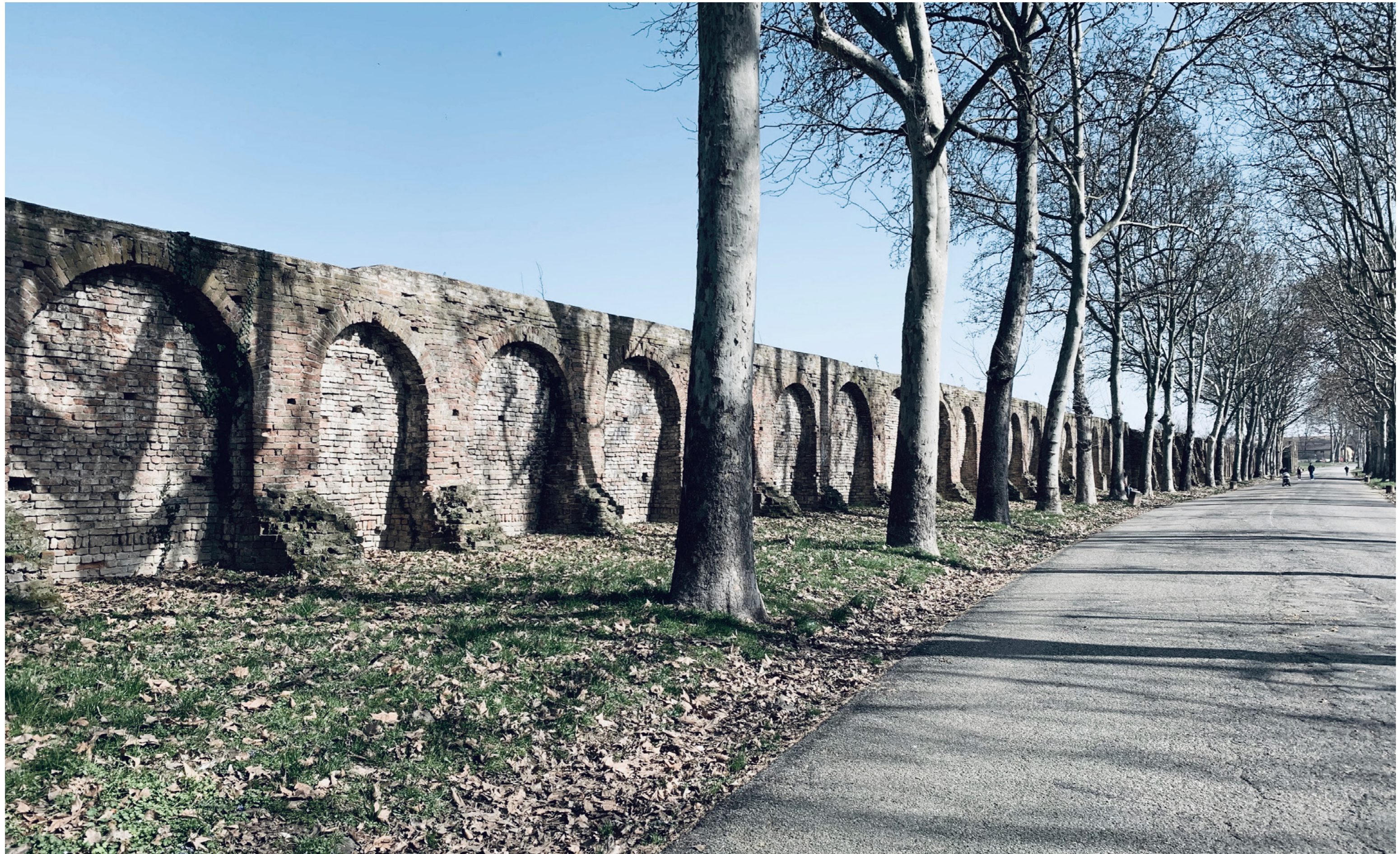
i The part of old wall in Piazzetta Borghetto
