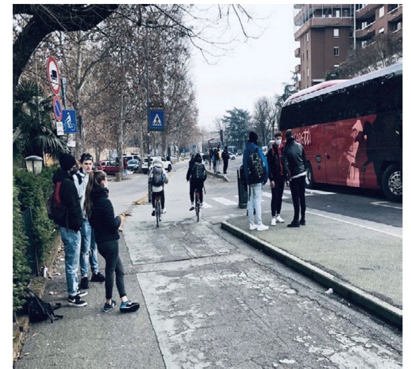
Lack of separation between users, damaged pavement
