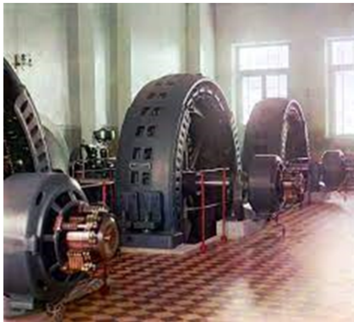
Figure 1.3: Power generator in a hydroelectric plant.
