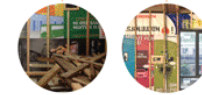
BATTENS FORMED FROM CUT DOWN SALVAGED PLY WASTE EXHIBITION BANNERS FORM VAPOUR CONTROL LAYER
