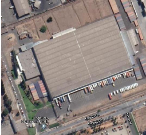
Figure 3-2: Satellite view of Johnson center.
