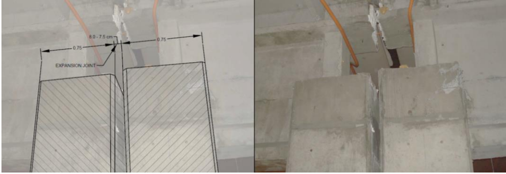
Figure 3-3: Expansion joint.
