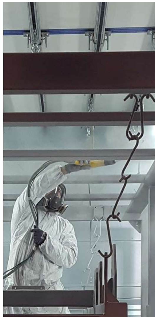
[1] painter reaching a difficult area
