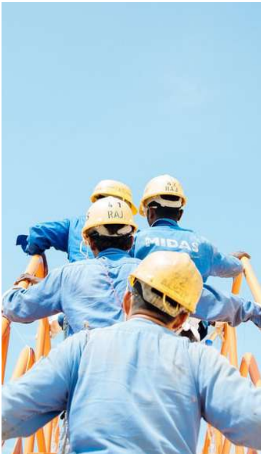
workers at work in a construction site
