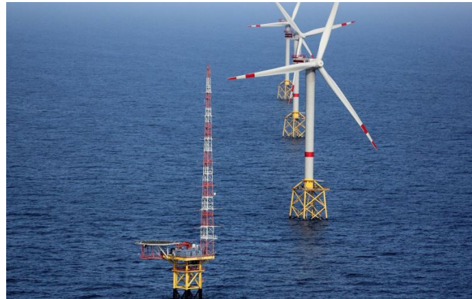
(b) FINO1 substation in front of Av04.
