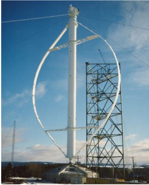
(a) The 110-m tall E'ole wind turbine, photographed in 1986
