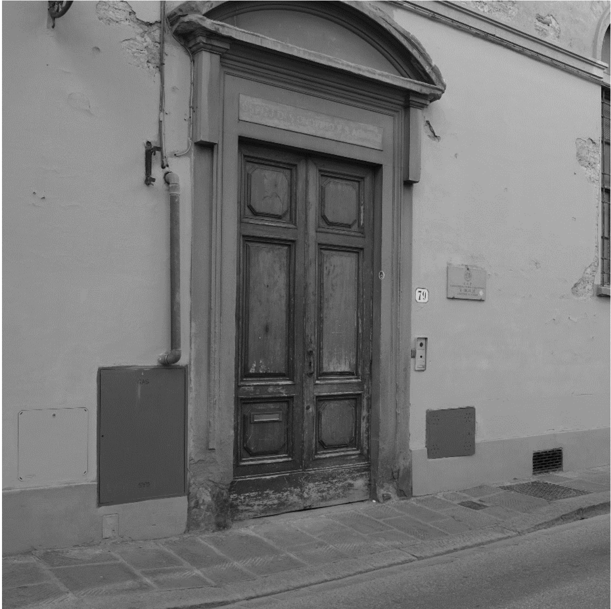
Figure 21 - Entrance to Via Guelfa 79 (personal shot, 2022)
