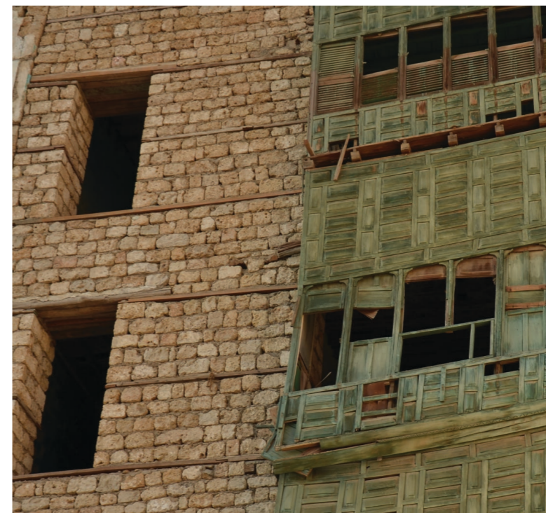
Figure88: An exposed wall on the right showing the coral stone and the Taklilas (Wooden Beams) every 5-6 rows of stone.
