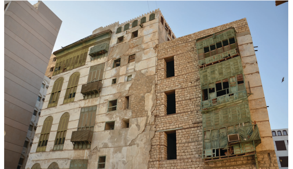
Figure88: An exposed wall on the right showing the coral stone and the Taklilas (Wooden Beams) every 5-6 rows of stone.
