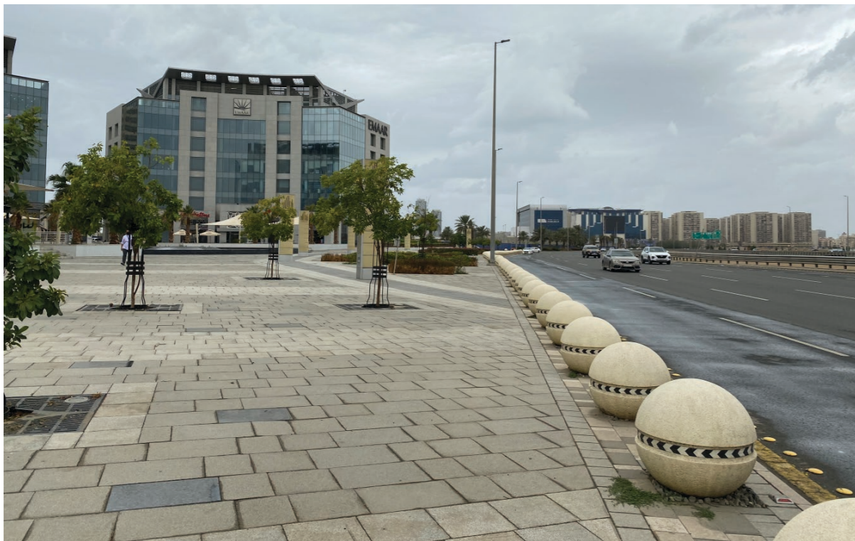
Figure96: The proximity of the high-speed road to the public space without a buffer zone is a source of noise and danger.
