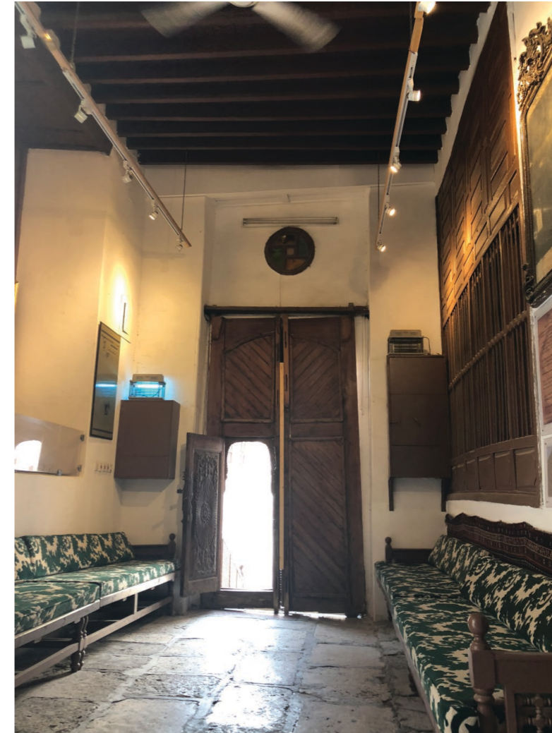
Figure91: The foyer of Ba'ishn House in Old Jeddah. The wooden ceiling was high enough to allow air circulation and aid in cooling the space. Fan and electric lights were added after renovation.
