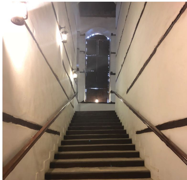
Figure90: The staircase of Nassif House. The staircase was wide and with low steps to allow the animals (horses or donkeys) to bring the groceries up to the kitchen, which was on the roof of the house for ventilation purposes. Wooden beams (Taklilas) show on the side walls as well.
