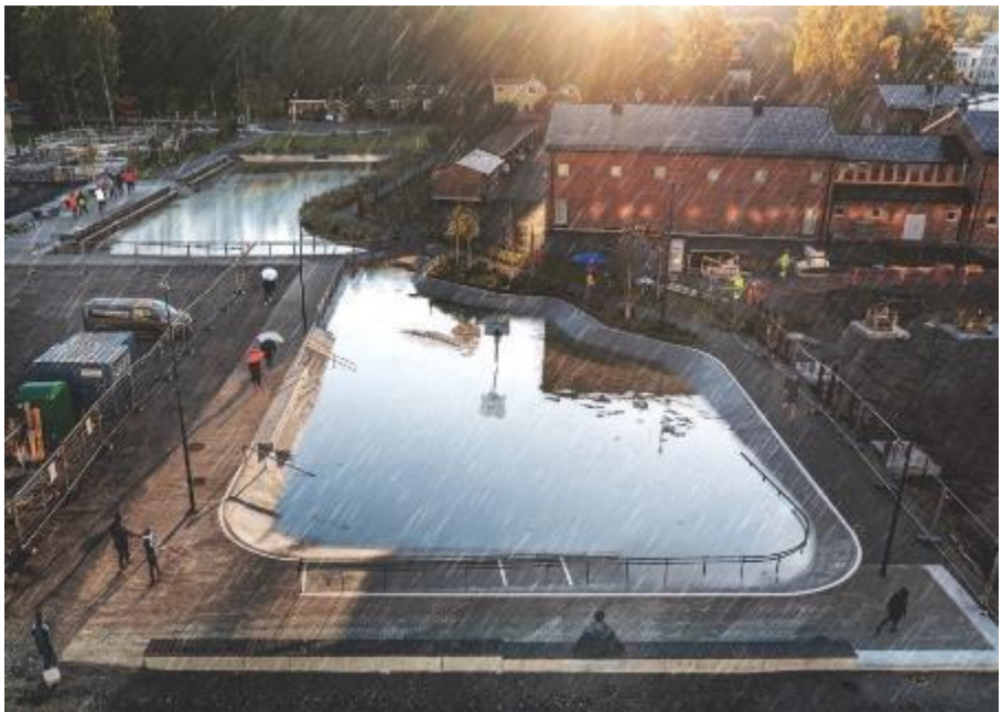
Figure 18 The skatepark during dry and wet conditions. Photo by Jann Lipka, simulation by Karavan landskapsarkitekter.
