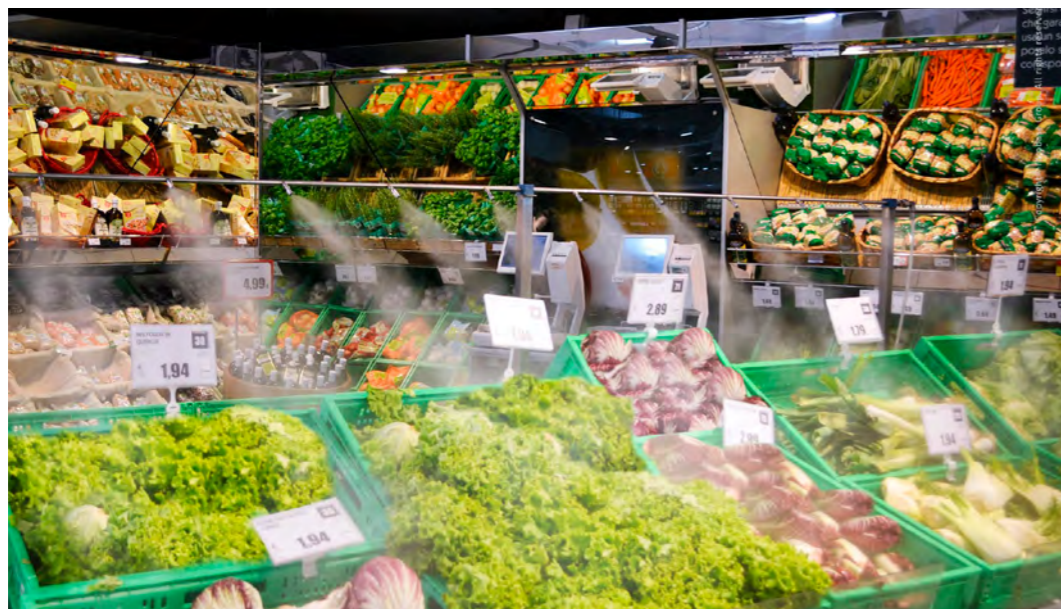
Fig.64 Preservation of fresh produce at supermarket, using ultrasonic humidification system.
