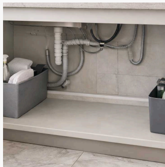
Under sink area
