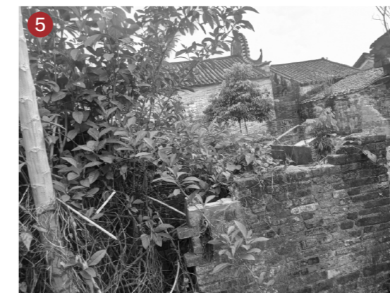
Plants grew into the interior of buildings, seriously affecting the use of the buildings
