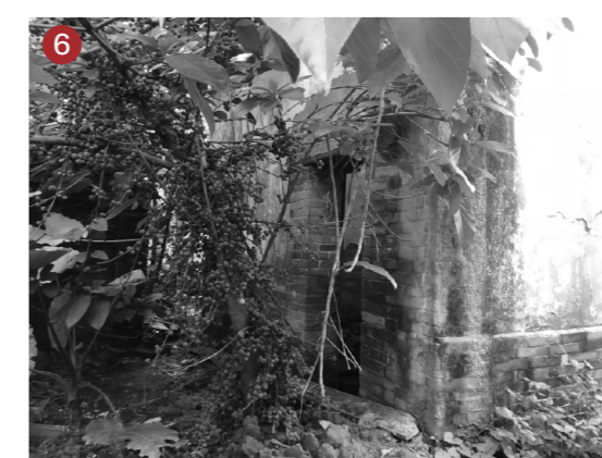
Plants left unattended, growing in entrances and exits of abandoned buildings.
