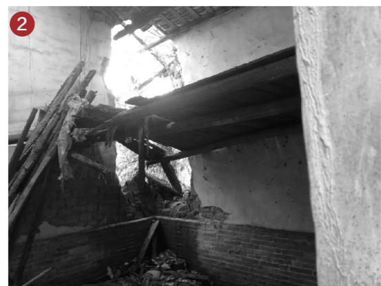
Part of the wall collapsed and the load-bearing structure of the building was damaged
