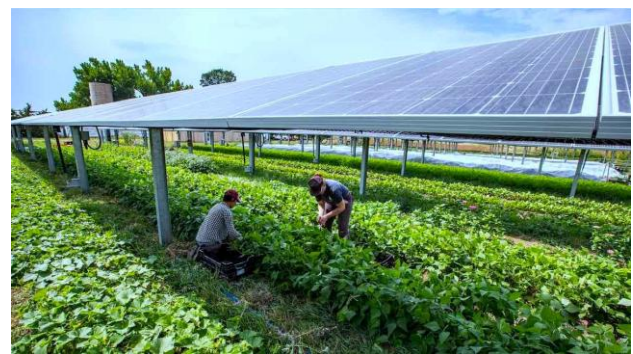
Figure 2.4: Fixed panels AVS [20]
