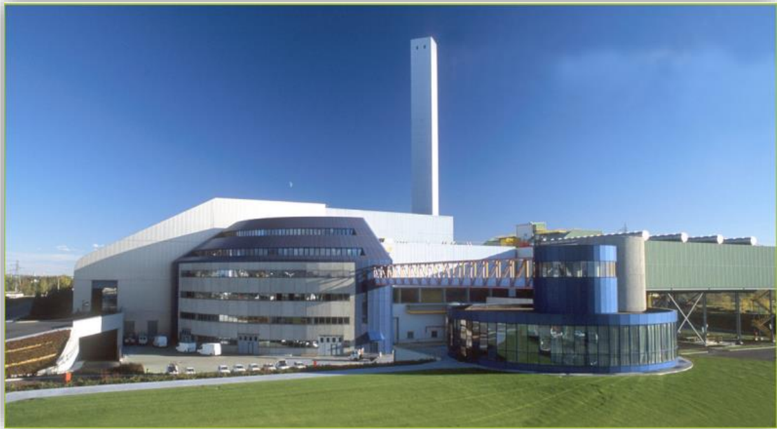
Figure 40 - Brescia Waste to Energy plant.
