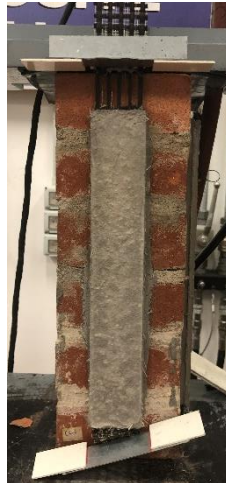
Figure 4-9: Failure developed in specimen DS_300_50_C_C_6
