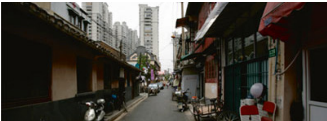
Figure 18, 19:: New and old urban fabrics in Lao-Cheng- Xiang are starkly juxtaposed (Courtesy of Hailin Zhai)
