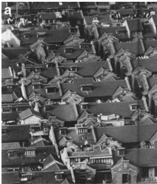
Figure 20: Rooftop scene of a Linong area. This widespread homogenous rooftop image is one of the most typical urbanscapes in central modern Shanghai. It is created by the repetition of a basic housing unit, a modified traditional Chinese town house, to form rows
