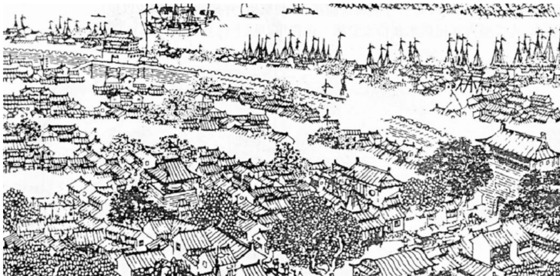
Figure 8: A view inside Shanghai walled city before the treat port time showing the typical structure of Chinese city with low-rise traditional courtyard houses, market, and street. Outside the wall were trading ports of this market
