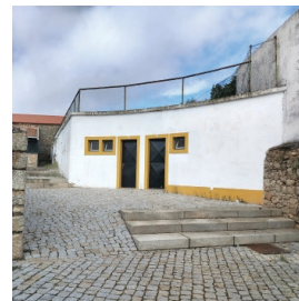
5b. Public toilets
