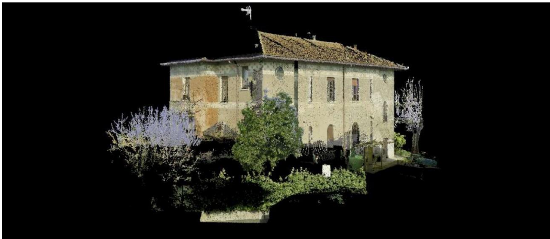
FIGURE 20- SOUTH VIEW OF CLEANED POINT CLOUD OF BUILDING TYPE A IN VIA SARCA 162
