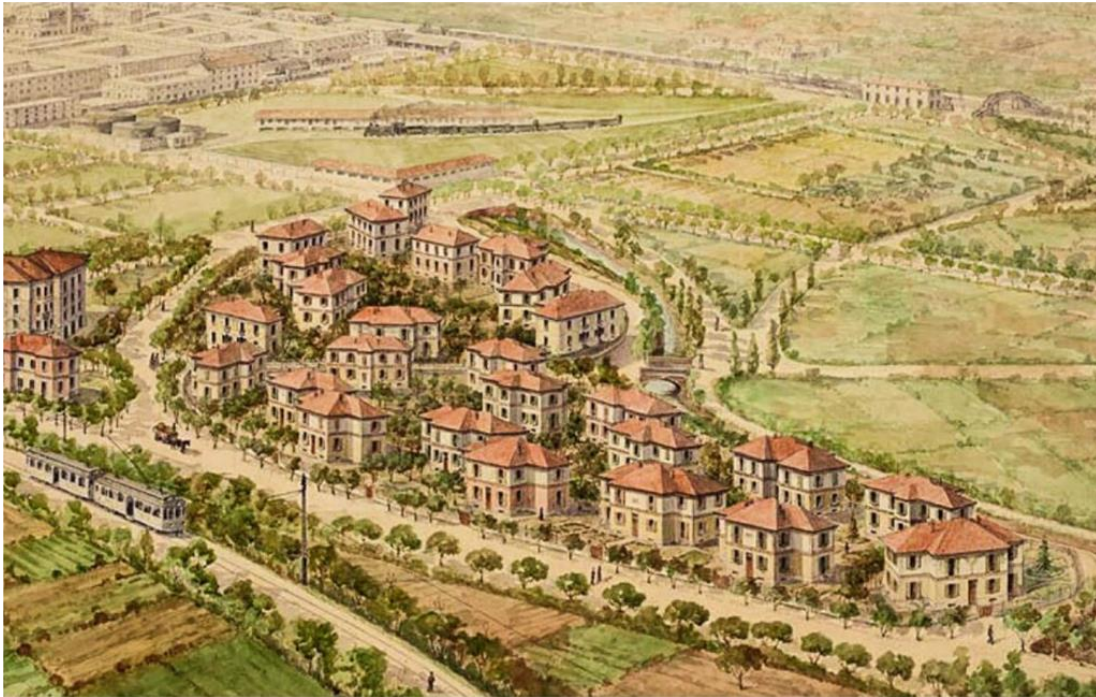
FIGURE 5: HISTORICAL PAINTING OF BORGO PIRELLI. THE BUILDING MODEL DEVELOPED RESEMBLES THE ROMANTIC SHAPE OF THE ENGLISH GARDEN CITY.
