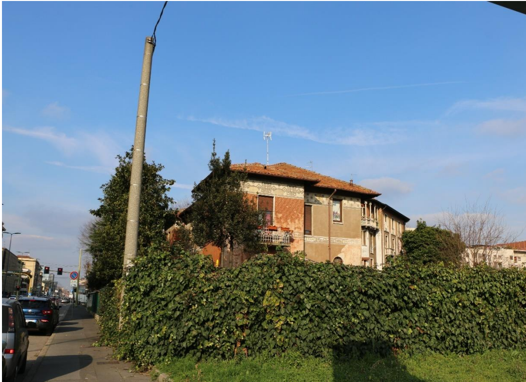
FIGURE 10: VILLA IN VIA SARCA 162 - BORGO PIRELLI-SOUTH VIEW
