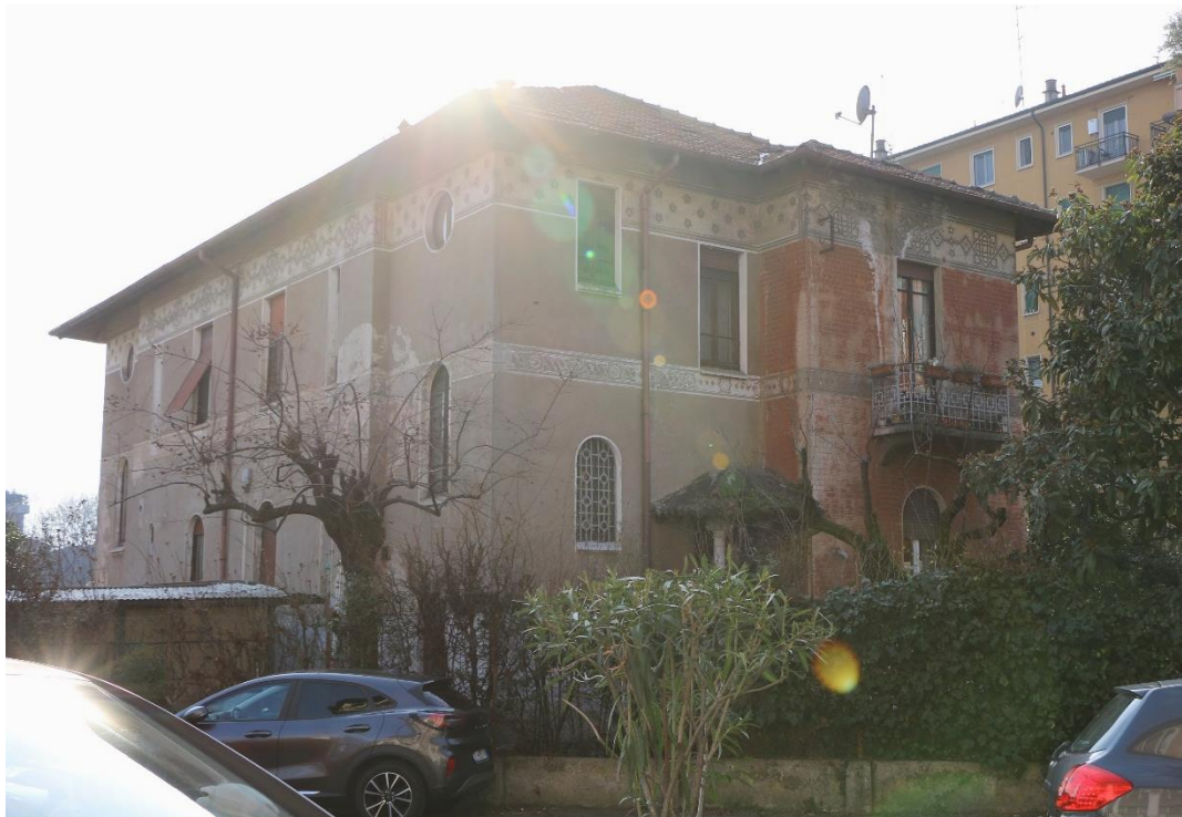
FIGURE 11: VILLA IN VIA SARCA 162 - BORGO PIRELLI-NORTH EAST VIEW
