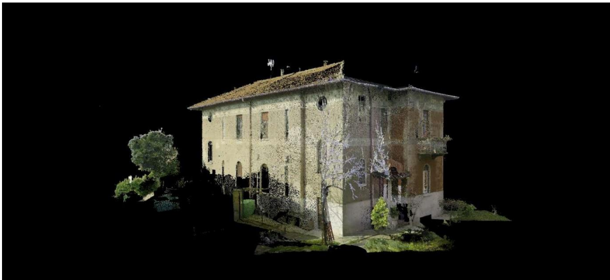
FIGURE 18- NORTH VIEW OF CLEANED POINT CLOUD OF BUILDING TYPE A IN VIA SARCA 162
