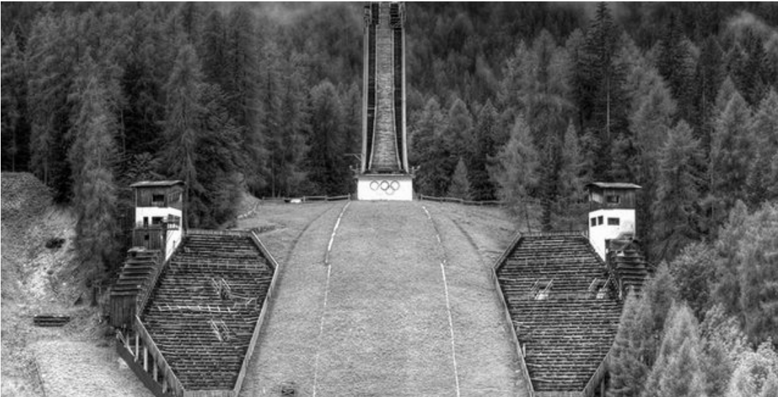
Fig. 58. Ski Jump Tower, Cortina D'Ampezzo, Italy, 1956 Winter Olympics Venue | Source: Google images
