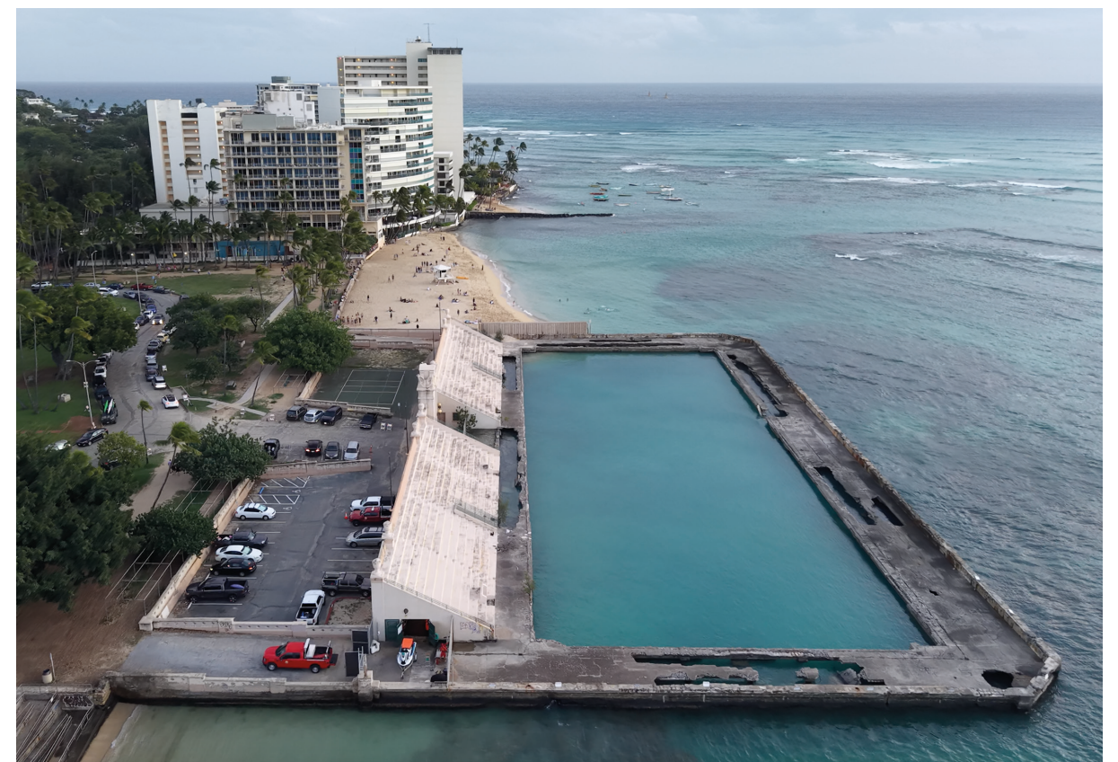
Fig. 25: Drone View of WWMN
