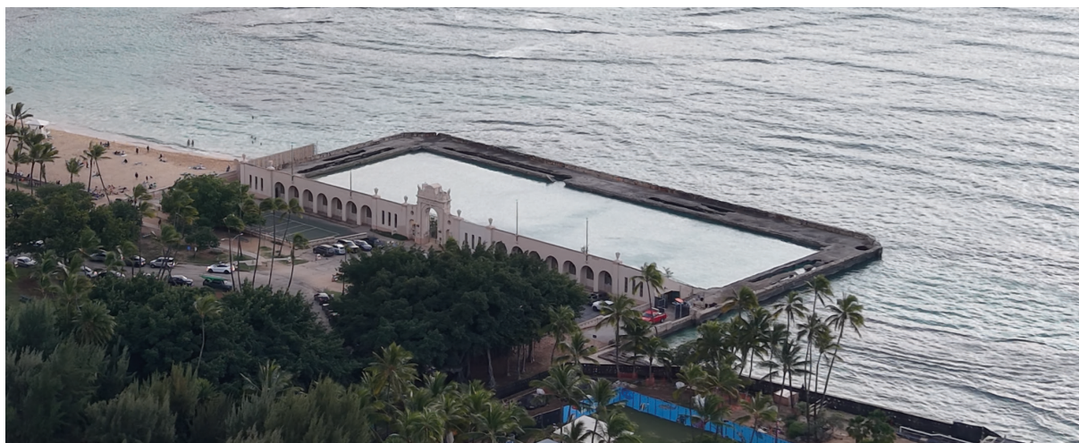
Fig. 24: Drone View of WWMN
