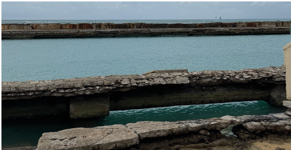
Fig. 33: Site-visit photo for perimeter condition 17.12.2025
