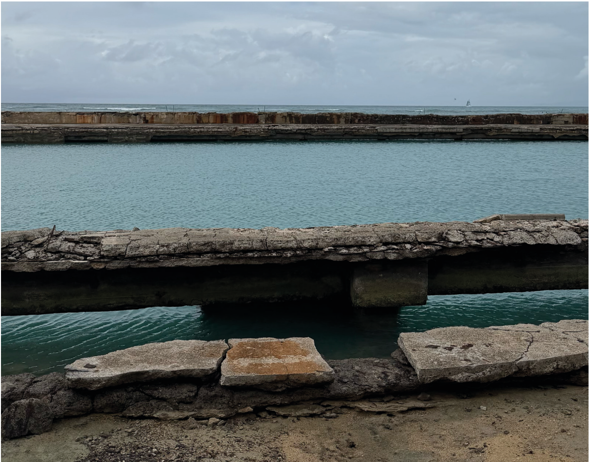
Fig. 06: Current Beams Situation Site-visit Photos December, 2025
