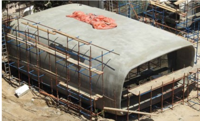
Figure 4: 3D printed office during applying the external finishing.
