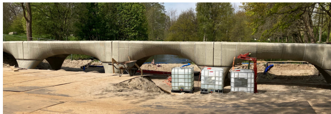
Figure 5: Assembly of the final bridge on location.
