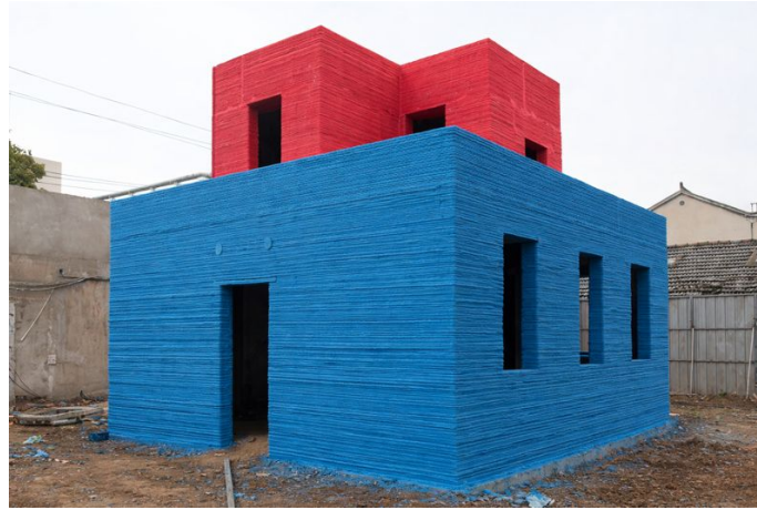
Figure 3: Panoramic photograph of the 3D printed two-story building.
