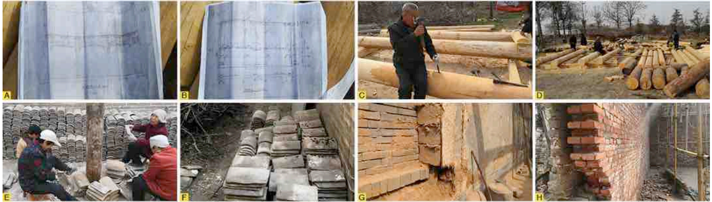
Figure 3-34 An example of reconstruction and restoration of a traditional courtyard house in Zhang-Dai-Cun Village. A,B - elevation and plan on which to rebuild the hall building; C,D - temporary site for wood processing outside the village; E,F - women clean up old tiles; G - traditional external blue brick wall and internal adobe bricks; H - in the hall building reconstruction project, modern red bricks are used instead of adobe bricks to be directly built on the inside of the old walls. Source: photos taken by the author.
