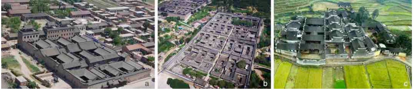
Figure 3-106 a. Cao's Grand Courtyard, Taigu, Shanxi Province; b. Wang's Grand Courtyard, Lingshi, Shanxi Province; c. Zhou's Grand Courtyard, Yongzhou, Hunan Province. Source: http://piao.wanbula.com/10209.html .; https://www.sohu.com/a/329455524_120028939 .; http://www.cnll.gov.cn/cnll/llfg/201511/a0c0446993d54fafa73950a84feb3da3.shtml .
