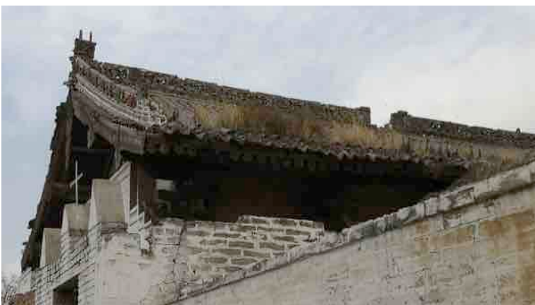
Figure 2-12 Yu Wang Temple in Shidai Village, Hancheng. The temple was built in the Yuan Dynasty (1271-1368), the exact age is unknown. In 1743 (eighth year of Qianlong in the Qing Dynasty) the temple was restored, and beams and purlins were replaced. It can be seen from the figure that the materials of the interior beams and purlins are different from the wood of the facade photo. (Photo by author).
