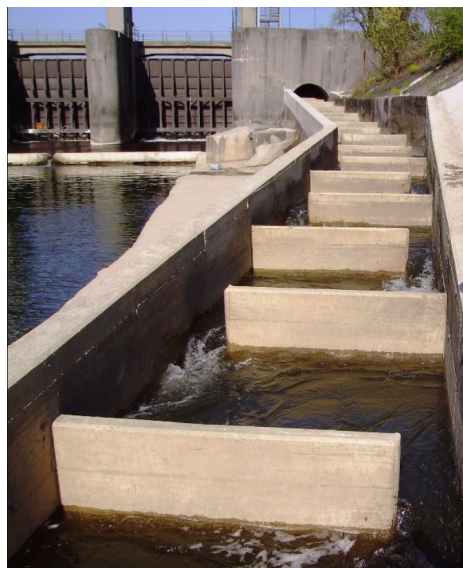
Figure 3.19: Sant'Anna dam, fish pool pass (Technical passage)
