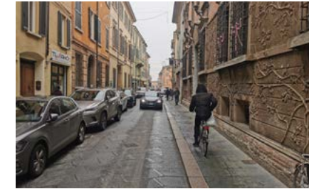
Poor safety for pedestrians and cyclists, light accidents are frequent
