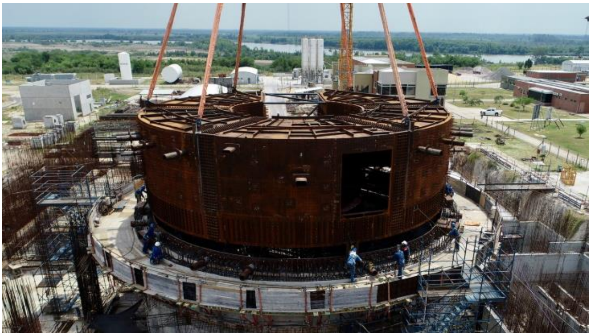
Figure 4 Installation of one containment liner module, CAREM (Source: CNEA)
