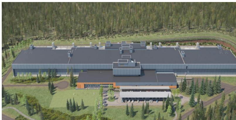
Figure 21. The Facebook data center in Lulea, Sweden (DataCenter Knowledge, s.d.)
