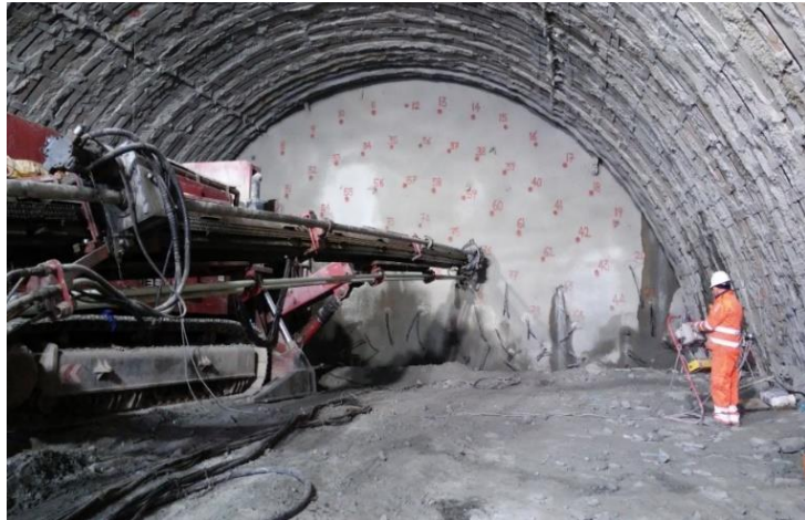
Figure 23 - VTR temporary structural elements disposal
