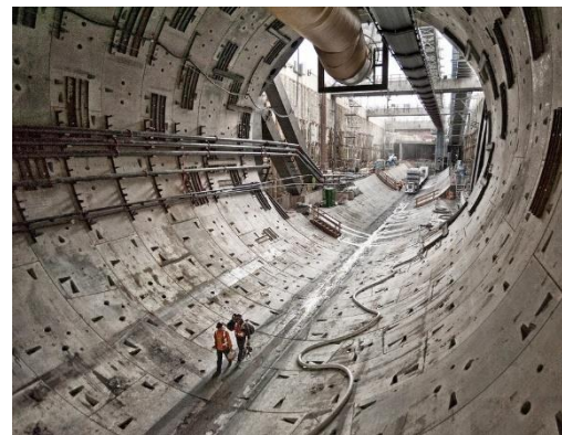
Figure 33 - Segmental TBM structural lining
