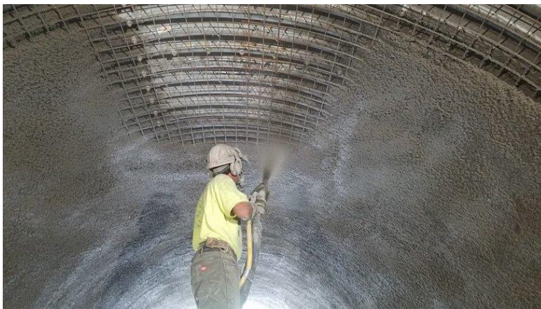
Figure 29 - Shotcrete layer disposal
