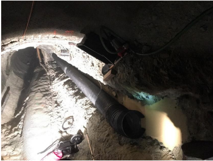
Figure 40 - Temporary drainage pipe functioning
