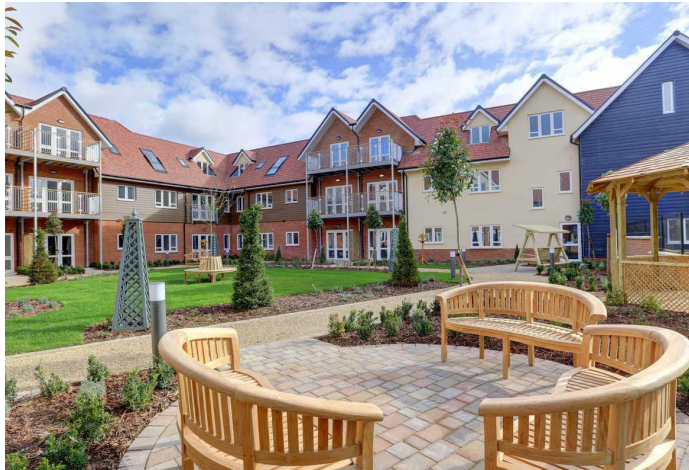
Figure 20. Retirement Housing Scheme, Anchor – Keble court, England
