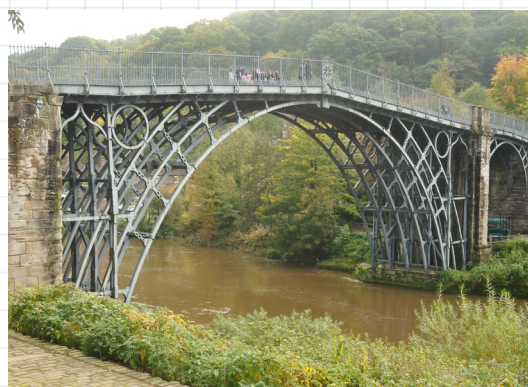
fig.2 Coalbrookdale Company Bridge, 1807
