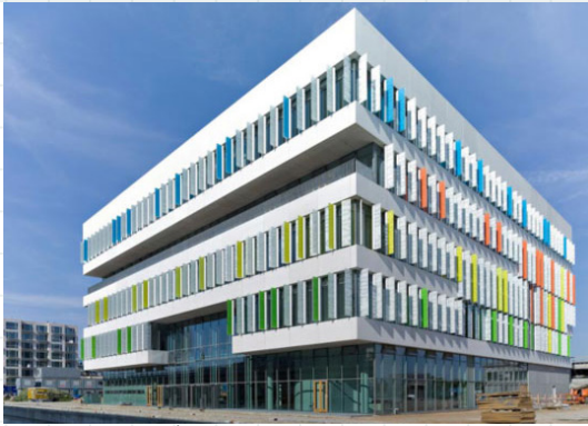
fig. 17. Vista esterna Ørestad Gymnasium School, Copenhagen
