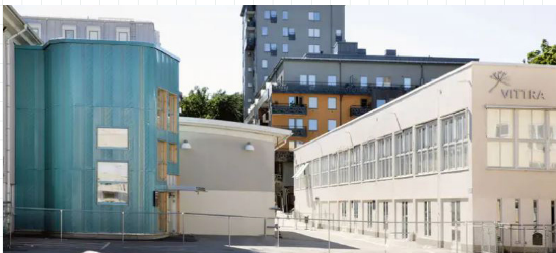
fig. 23 Vista esterna Telefonplan Vittra School, Stoccolma
