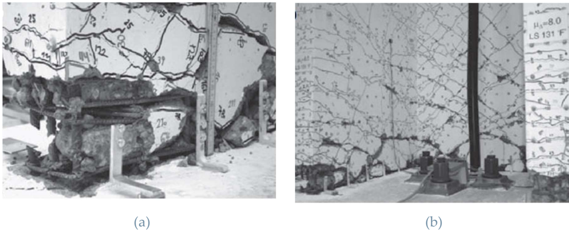
Figure 2.7 Failure of TUA (Beyer et al., 2008b)
