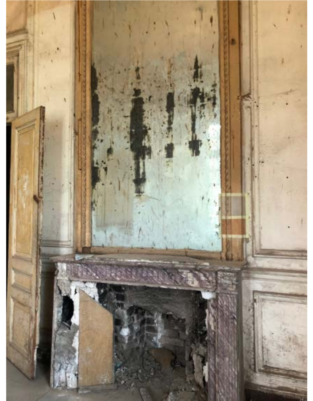
Damages to the Marble Fire Place
